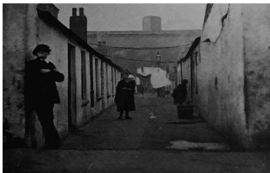
Brady's Cottages (off Townsend Street).
