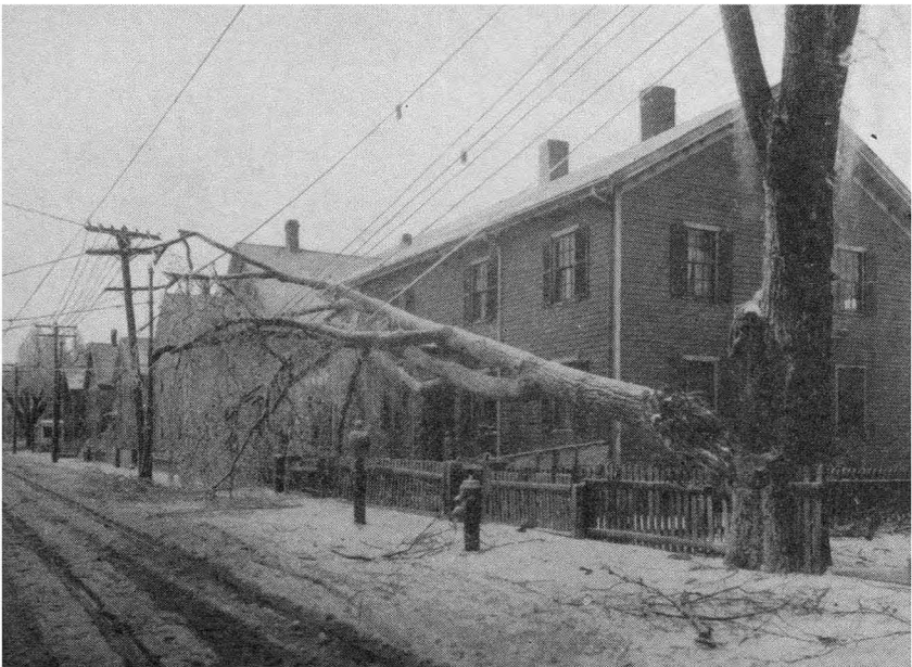
Figure 2. Advanced decay in this elm and a sleet storm combined to interrupt wire service in this community. Damage by this fallen tree could have been even more serious; note proximity of dwelling house and police and fire equipment. Photograph furnished by Boston Edison Co.
