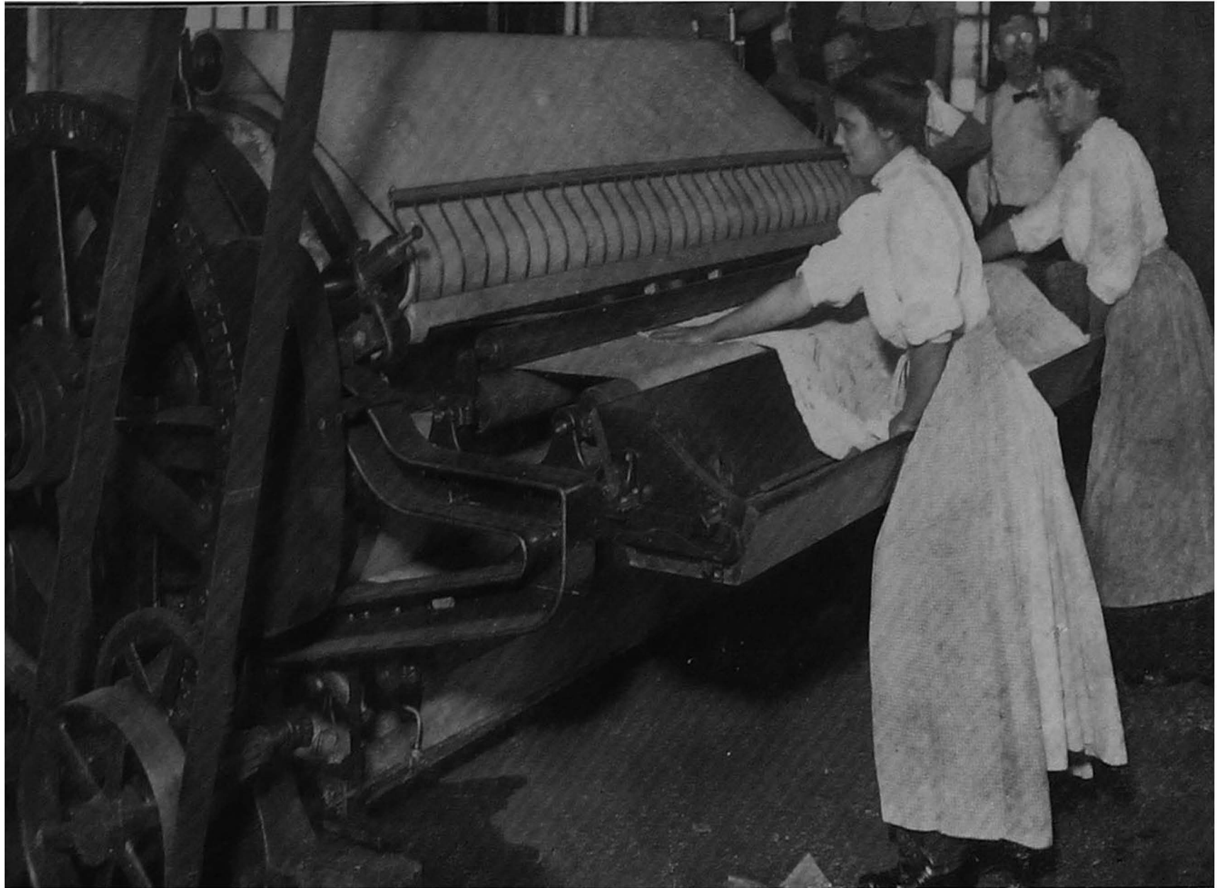
THE FEEDER AT A CYLINDER MANGLE.
