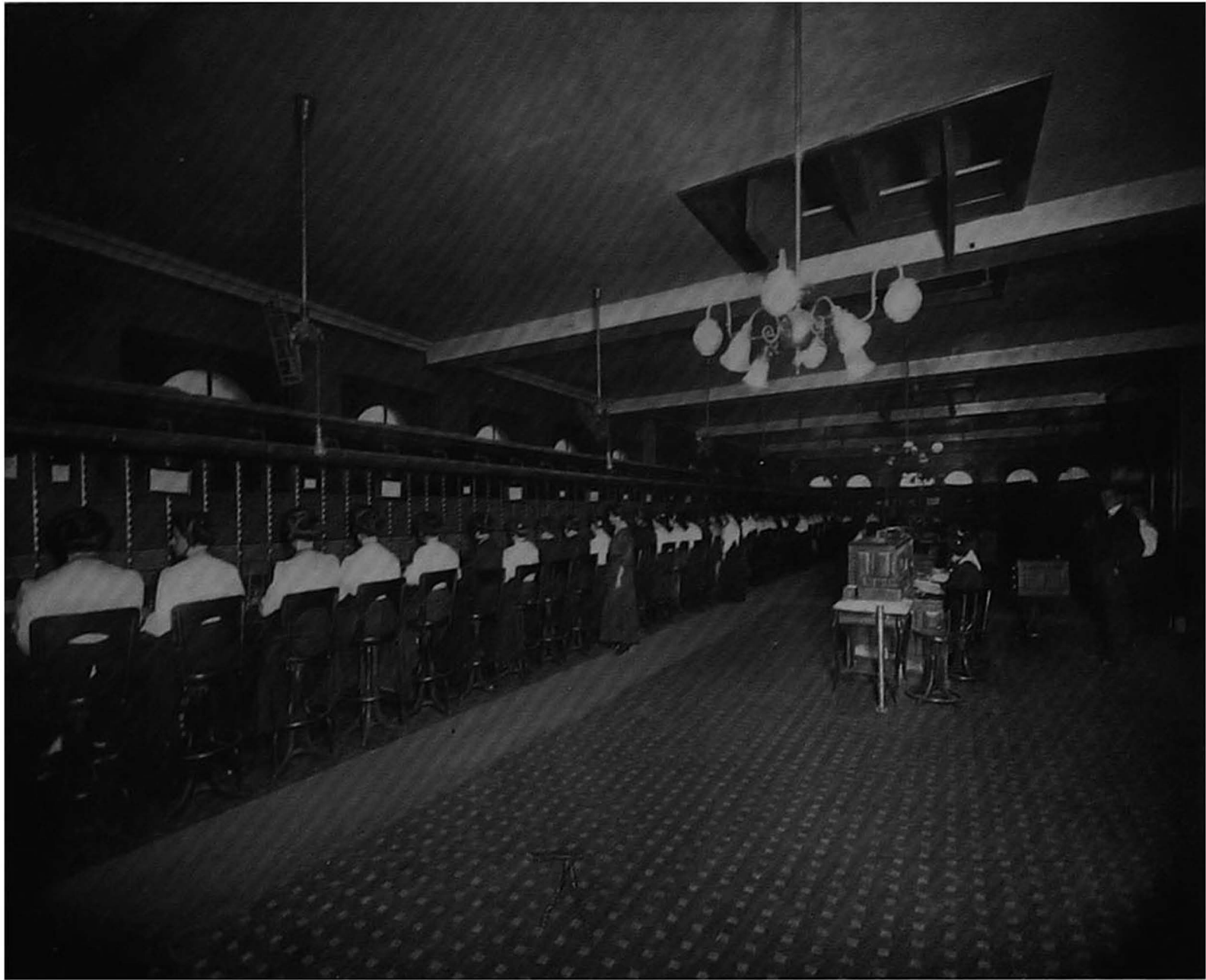
A TELEPHONE EXCHANGE
