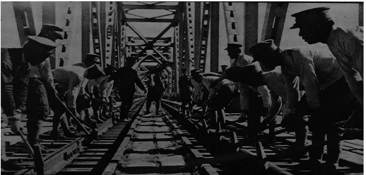
Changing the Gauge of the Hsinking-Harbin Line
