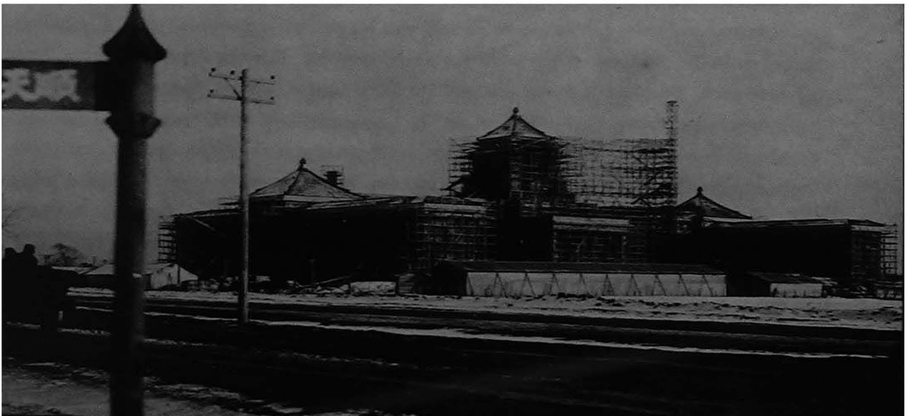
New Hsinking: The State Council Building under Construction
