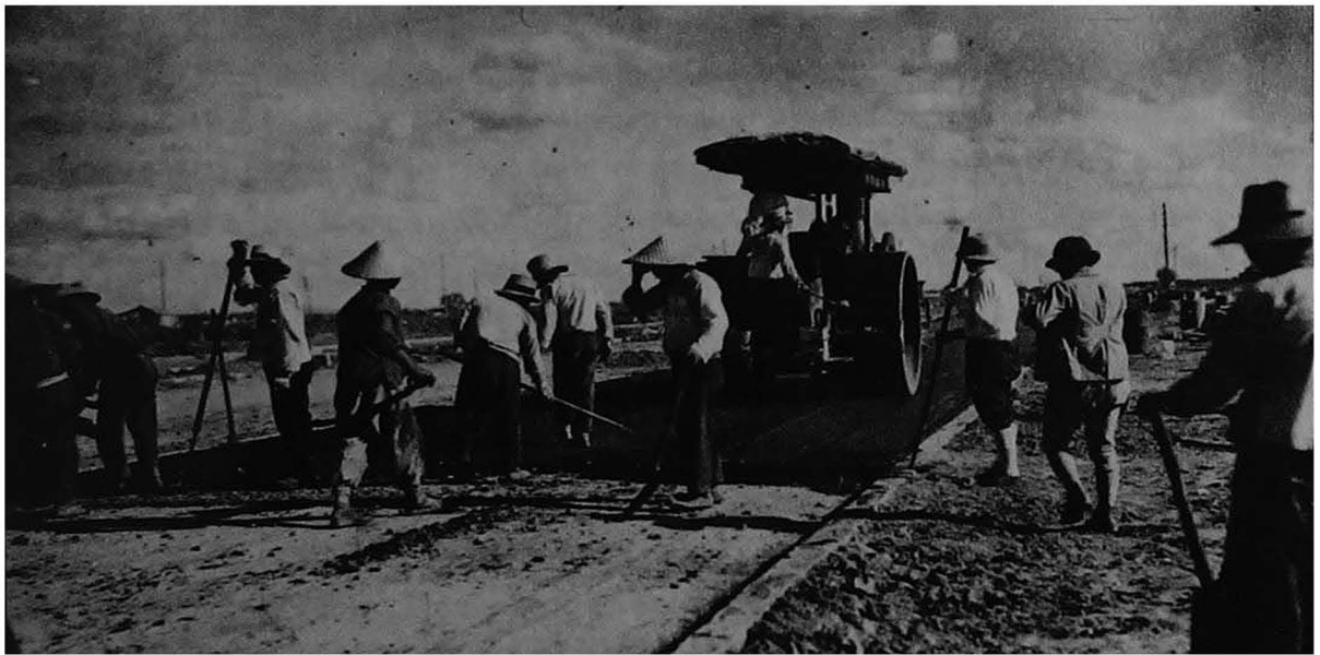
A Scene of the Highway Construction Work
