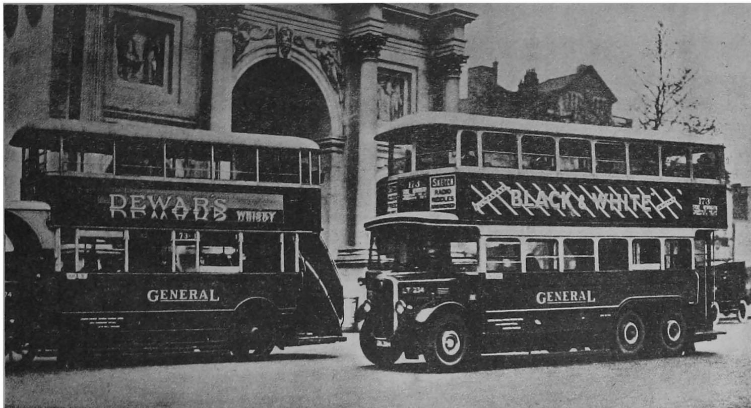
LONDON'S BUSES, SIX- AND FOUR-WHEELED, BUT BOTH WITH THE ENCLOSED UPPER DECK THAT HAS NOW BECOME THE STANDARD THING FOR CITY TRAFFIC
