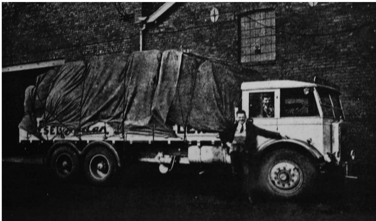
THE FODEN-DIESEL SIX-CYLINDER 10-12 TON SIX-WHEELER WITH A GOOD LOAD (By courtesy of Fodens, Ltd.)
