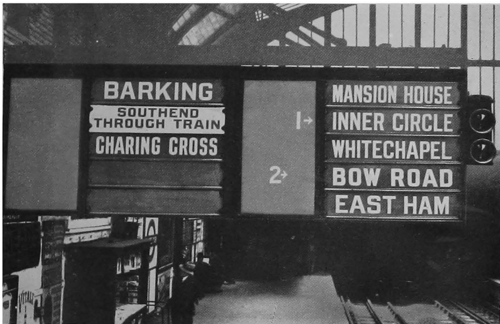
Fig. 47. Another type of platform train indicator (District Line).
