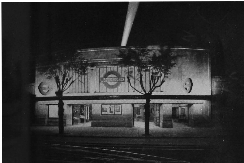
Fig. 118. Tooting Broadway Station, City and South London Railway, showing the striking effect of flood-lighting. The beam of a searchlight can be seen above the roof.
