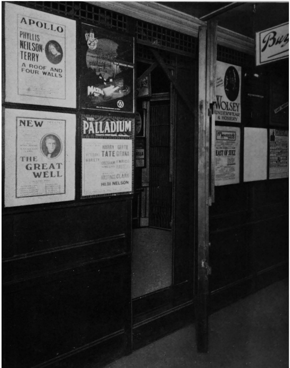
Fig. 63. The emergency door, by means of which passengers in a disabled lift can gain access to an adjacent one and thus continue their journey.
