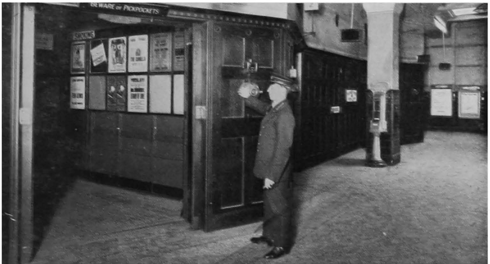
Fig. 62. A lift being manipulated by means of the landing control equipment.
