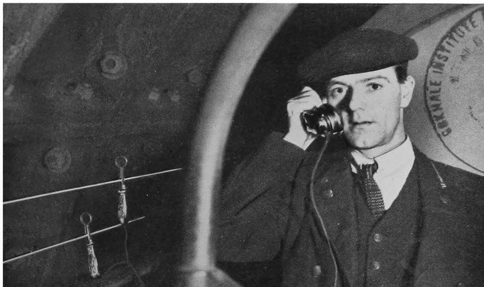
Fig. 49. A driver using his portable telephone set. By hooking the terminals to the bare wires in the tunnels he is enabled to communicate with the sub-station.
