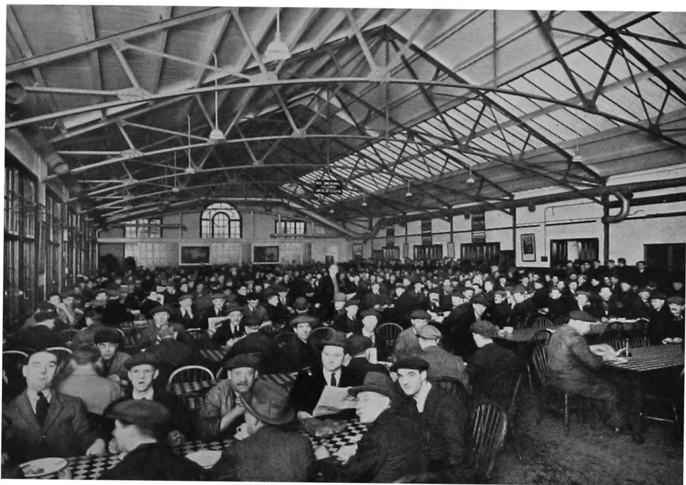
Fig. 131. One of the messrooms for employees.
