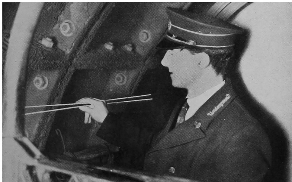
Fig. 50. The action of pinching the wires in the tunnel, as shown, enables the train-man, in emergency, automatically to operate the sub-station cut-out.
