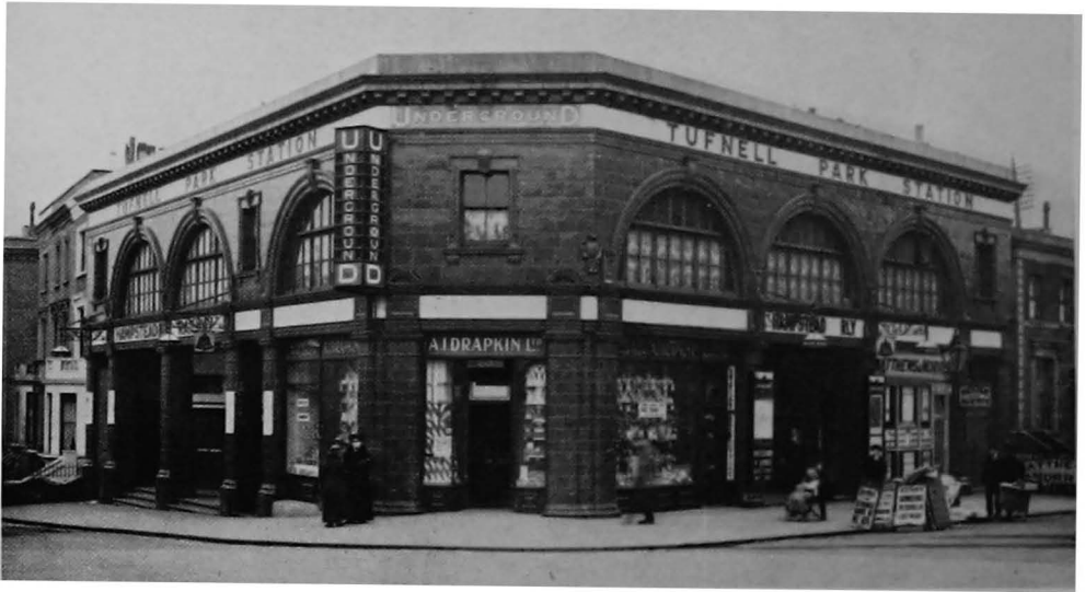
Fig. 121. One of the original London Electric Railway stations.
