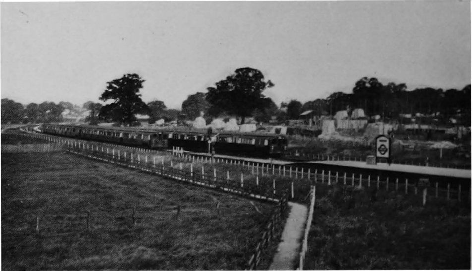
Fig. 141. Burnt Oak Station on the Edgware Extension of the Hampstead Railway, showing houses in course of erection.
