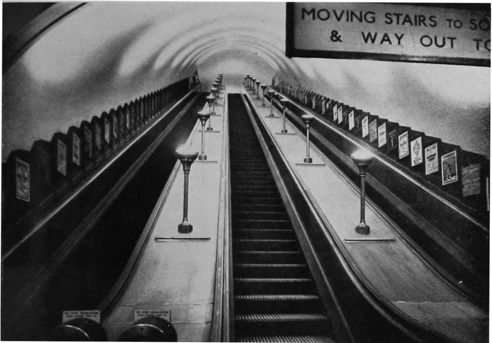
Fig. 127. A set of the latest type escalators.
