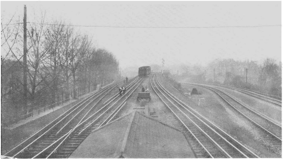
Fig. 35. 'Flying' junction west of Turnham Green, looking west.
