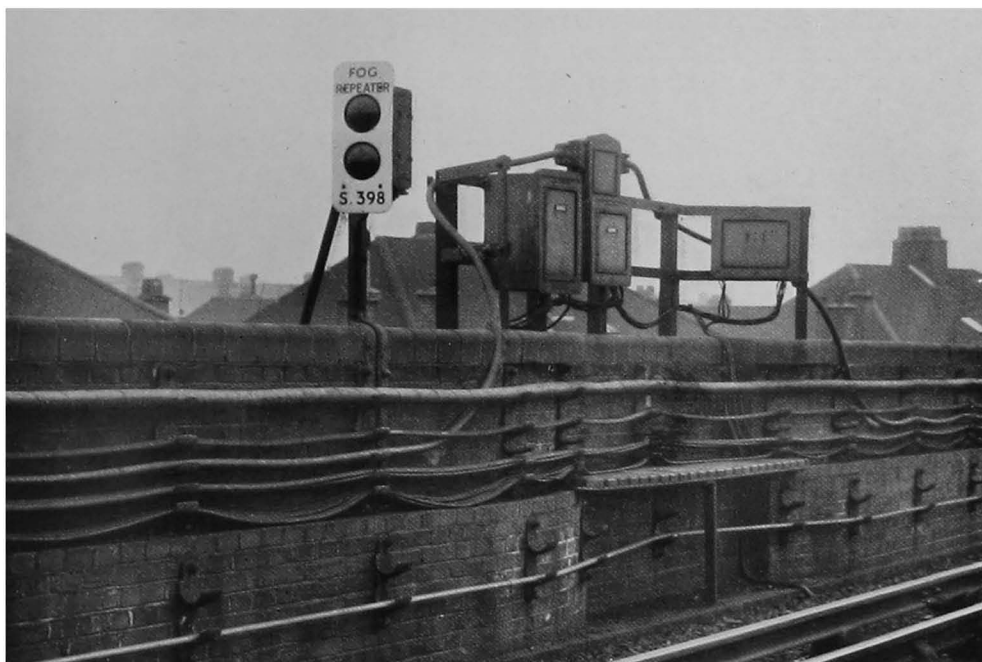
Fig. 45. A typical fog-repeater signal.
