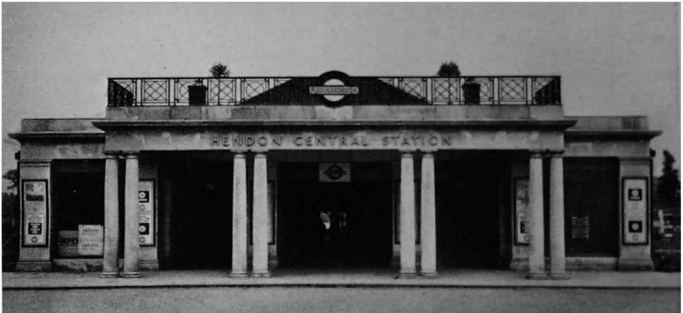
Fig. 119. Hendon Central Station on the Edgware Extension of the Hampstead Railway.
