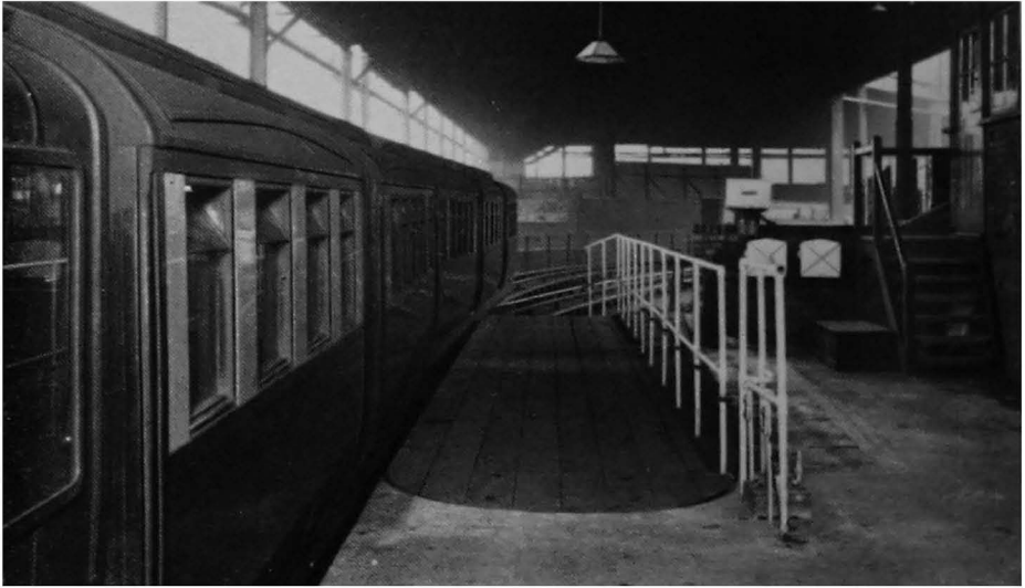
Fig. 126. The movable platform extension at Wood Lane.
