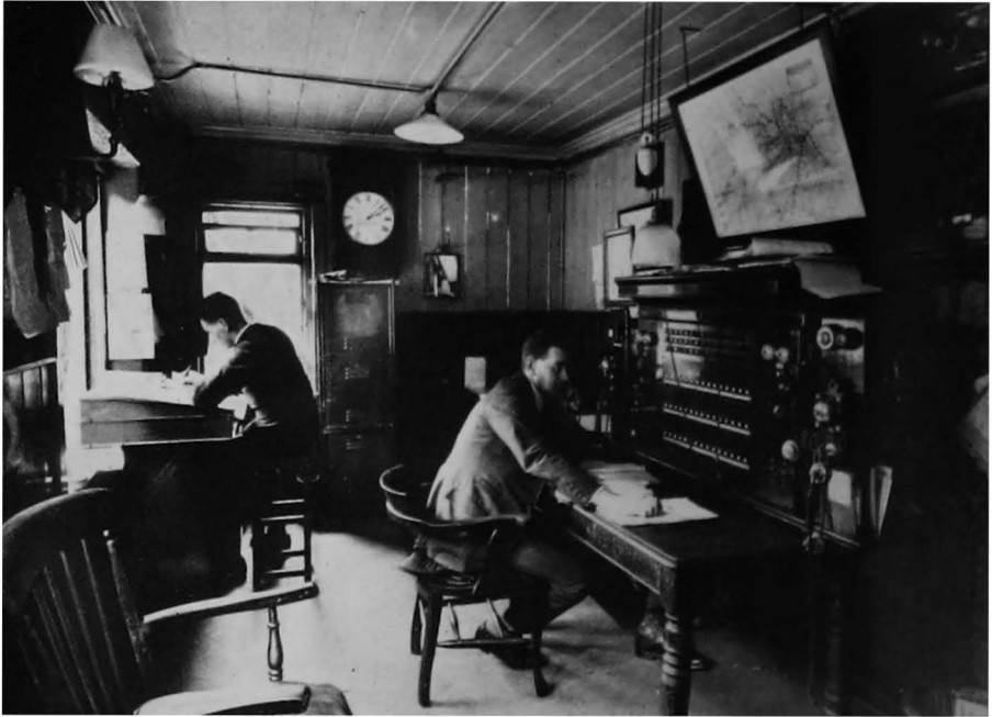
Fig. 37. District Railway control office, Earl's Court.
