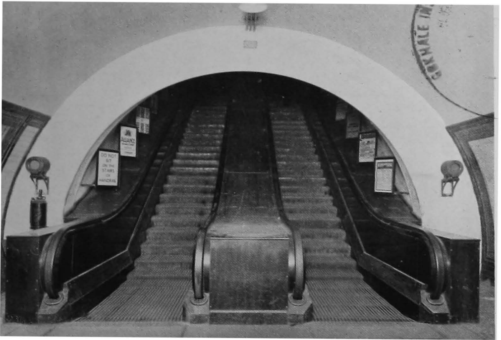
Fig. 129. Comb-type escalators.
