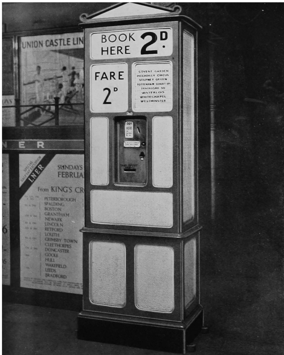
Fig. 102. Standard type of automatic ticket-issuing machine.
