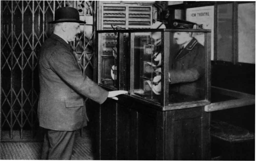
Fig. 113. A lift equipped with a pedestal booking-booth, an arrangement in operation at some of the less busy stations.
