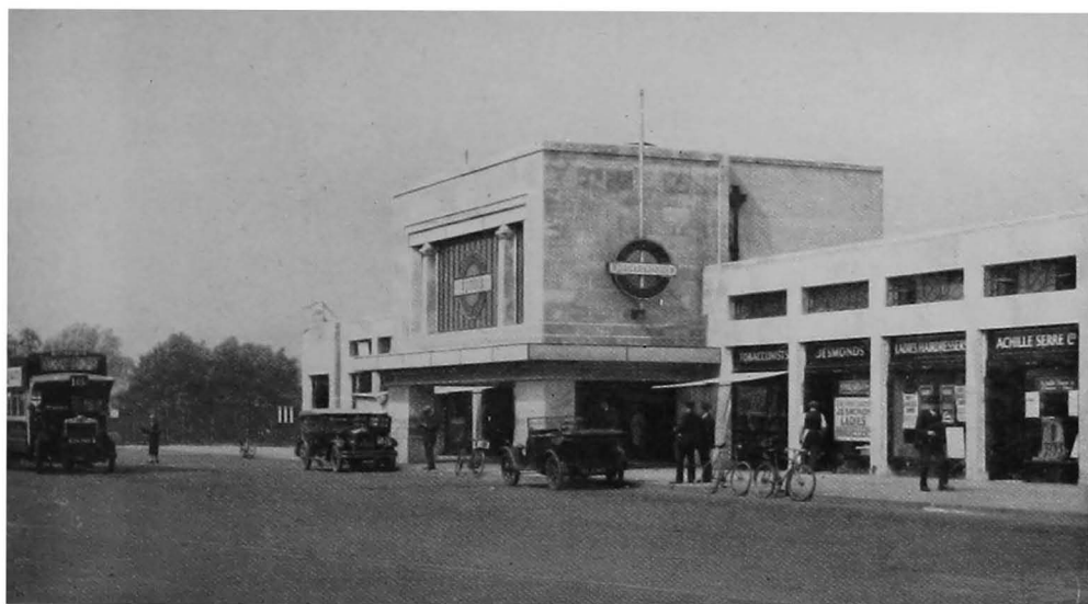
Fig. 116. A new station on the Morden Extension of the City and South London Railway.
