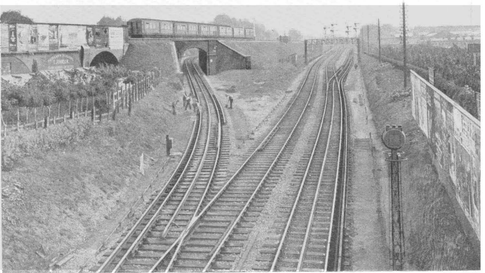
Fig. 36. 'Flying' junction at Turnham Green, looking east, showing the 'up' Richmond line passing under the main line.
