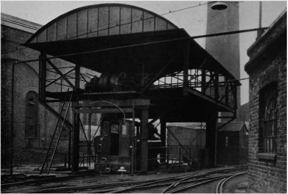
Fig. 90. The 20-ton hydraulic lift which was used at Stockwell to raise locomotives and coaches from the railway below preparatory to their undergoing repairs in the shops. The appliance proved invaluable during the subsequent reconstruction of the railway.
