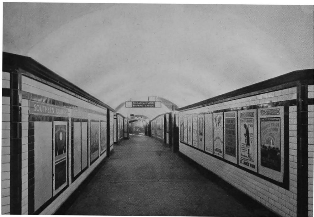
Fig. 122. A subway at Finsbury Park Station, showing the effect of flood-lighting as applied to interiors.
