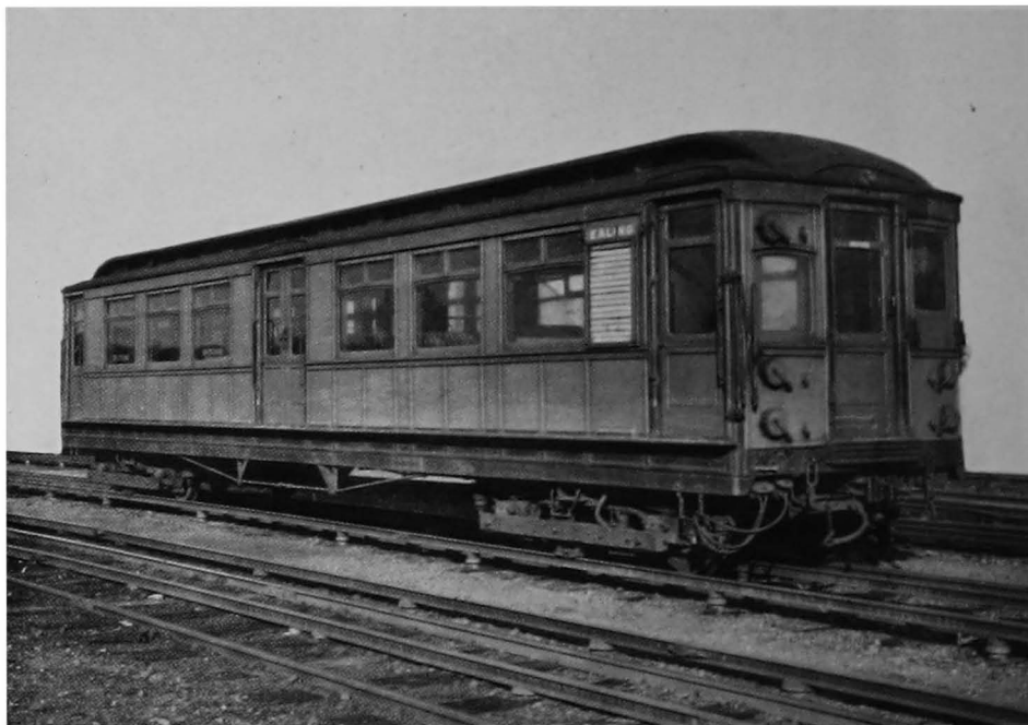
Fig. 78. District Railway coach, in service immediately after electrification.
