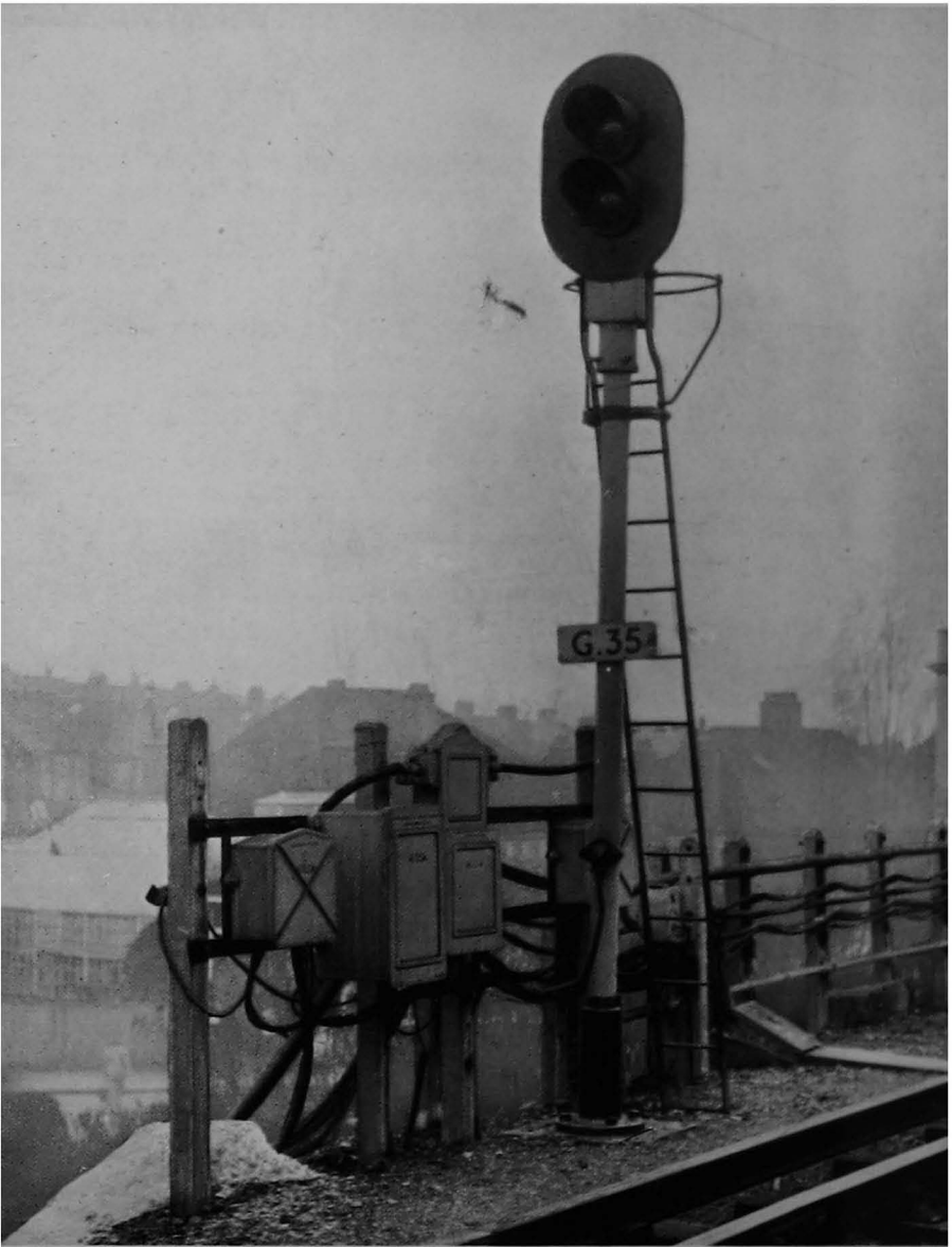
Fig. 44. Two-position day colour light signal.
