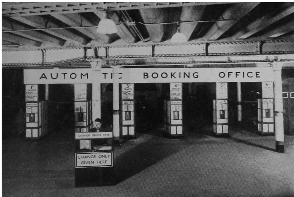
Fig. 112. The automatic booking-hall at Bank Station; note the change-giving booth in the foreground.
