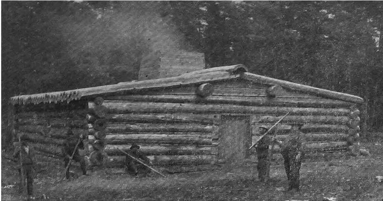
SHOWING THE FRAMED CHIMNEY, THE CHINKED WALLS, AND COMMON MODE OF ROOFING This particular shanty was specially constructed in 1900 for demonstration purposes, consequently it is superior to the average shanty formerly built on isolated works
