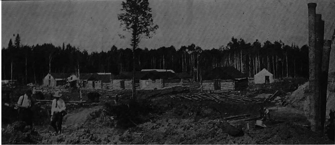
BUILDINGS SHOWN: A. WAREHOUSE; B. OFFICE; C. FOREMEN'S BUNKHOUSE; D. COOKERY; E. MEN'S BUNKHOUSE
