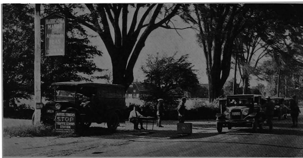
One of the traffic survey stations on U. S. 3, the Daniel Webster Highway. This was both a recording and weighing station
