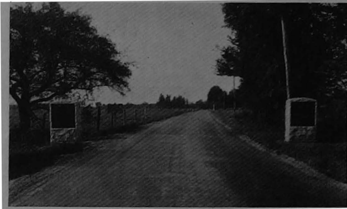
Bituminous macadam surface on Route 10. Note Dartmouth College road markers
