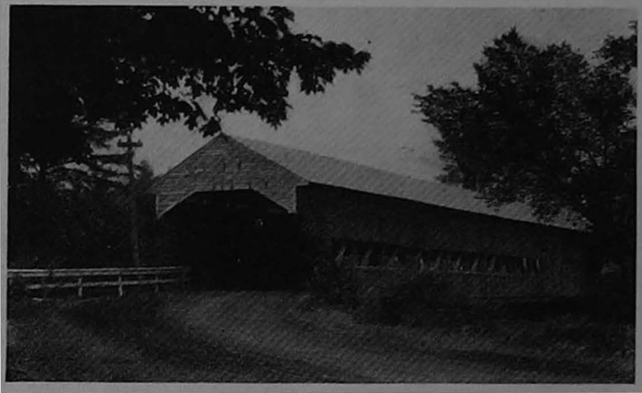
An old covered bridge. Many of the older bridges are no longer adequate and will have to be replaced
