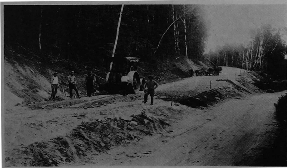
Relocating a highway which is to be gravel surfaced, near Newburg
