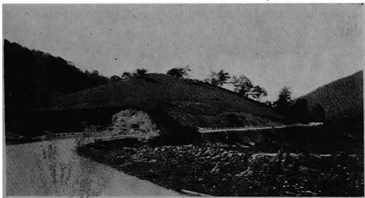
The State Road between Sherburne and West Bridgewater in Rutland County, improved with Federal aid as a gravel road
