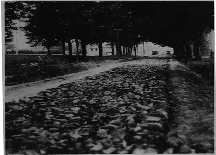
A stone base under construction north of St. Albans
