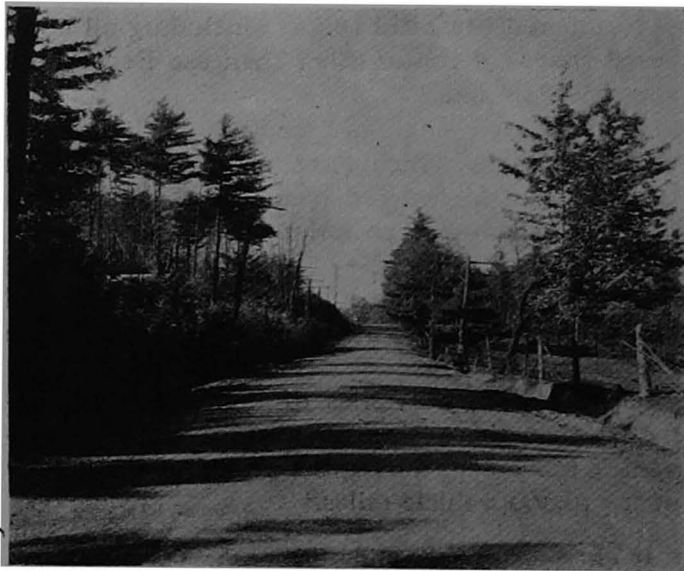
Federal-aid Project No. 13, near Addison, a bituminous macadam road
