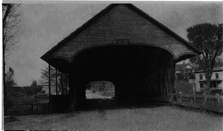
A covered 2-way wooden bridge over the Passumpsic River near St. Johnsbury
