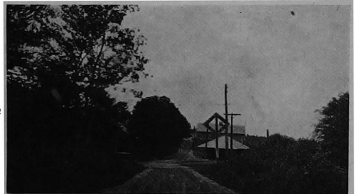
A dangerous railroad grade crossing eliminated by the construction of Federal-aid Project No. 58, an improvement of the Summit Road between Gassetts and North Clarendon. The new road is surfaced with gravel.
