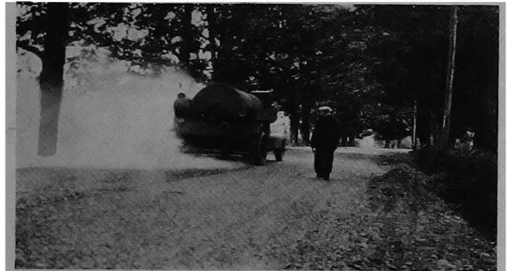
Applying seal coat on the Bernardstown Road
