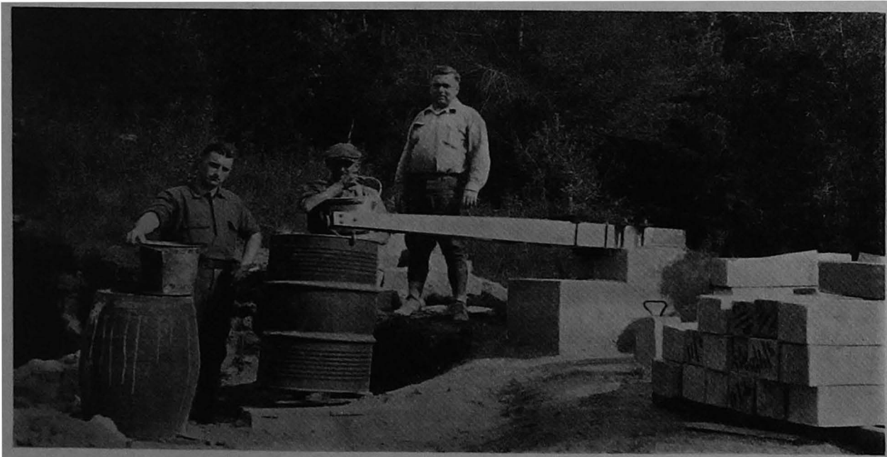
Testing specimens of concrete in the field as a means of controlling the strength of concrete pavements
