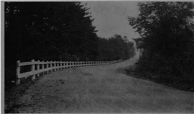
The River Road between Farley and Bradford—a gravel road constructed with Federal aid
