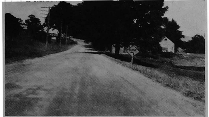
U. S. Route No. 5, near Hartland. The road is surfaced with gravel. Note the standard caution sign
