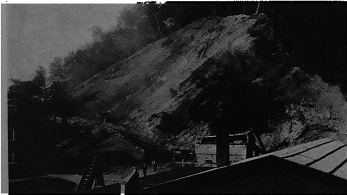
The gravel bank from which material was taken for the construction of Federal-aid Project No. 91A, near Hartford
