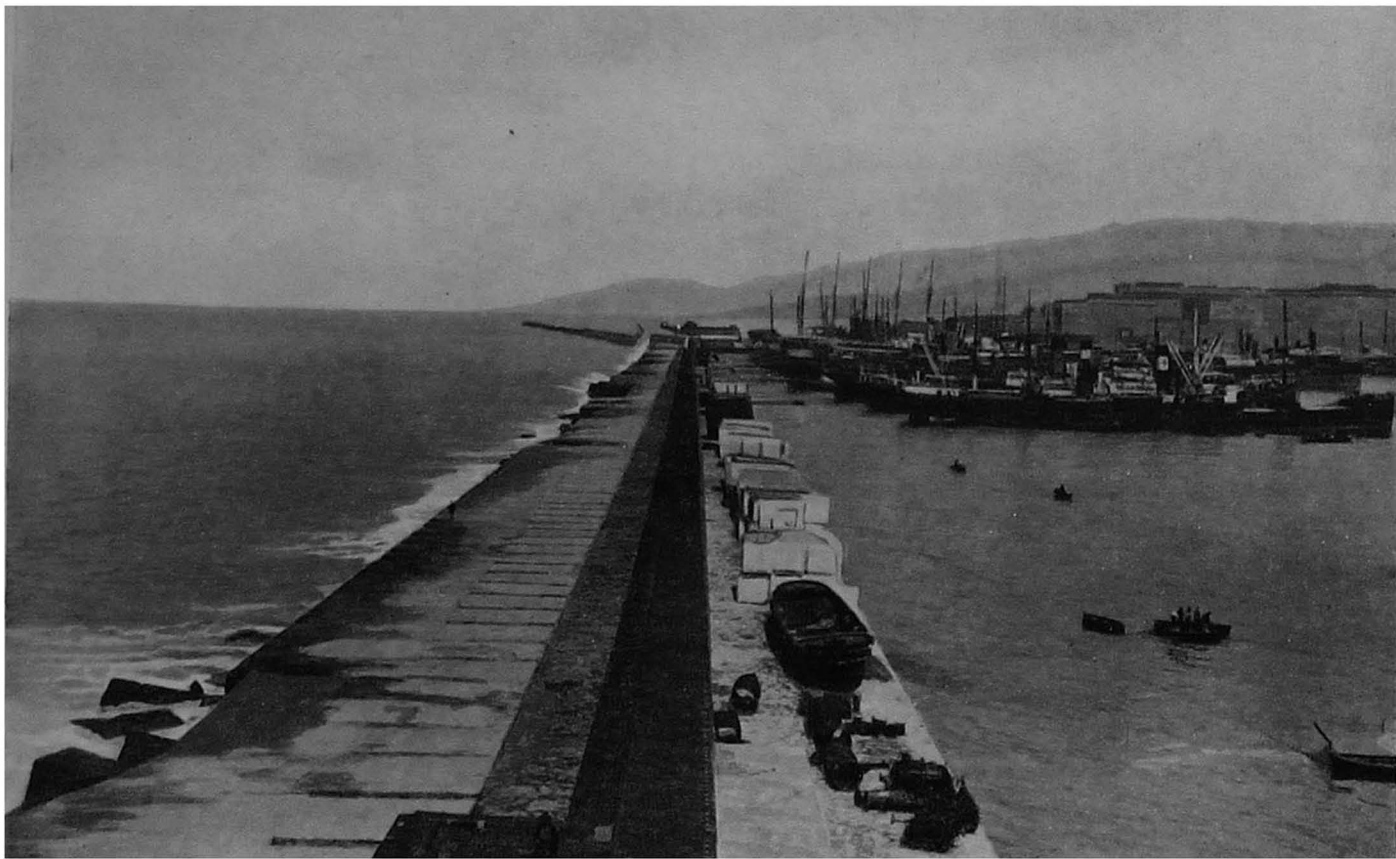
The Galliera Mole, Genoa. (Artificial protection across the front of the harbour.)
