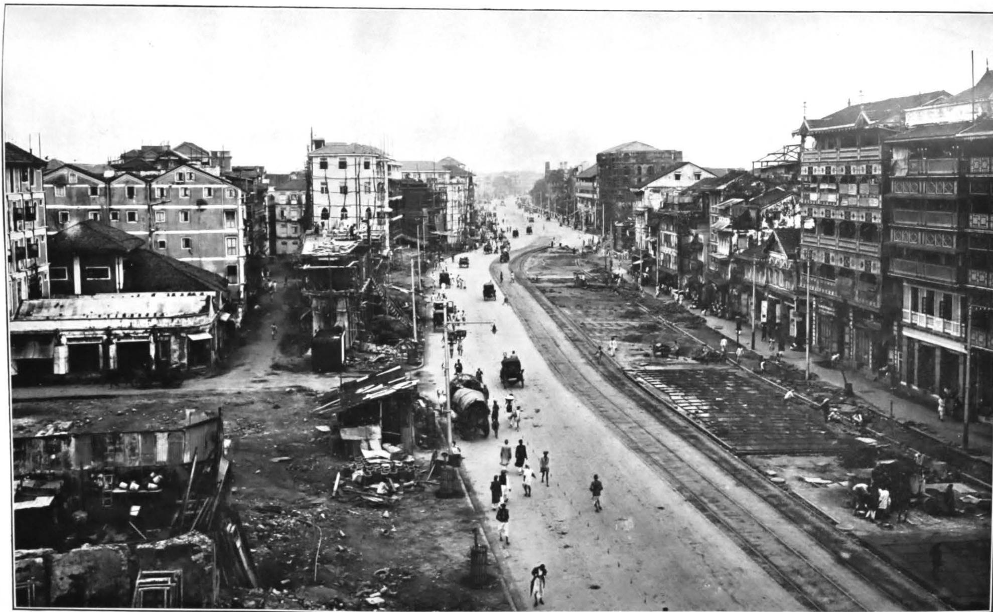
Parel Road under construction looking North from Sandhurst Road.
