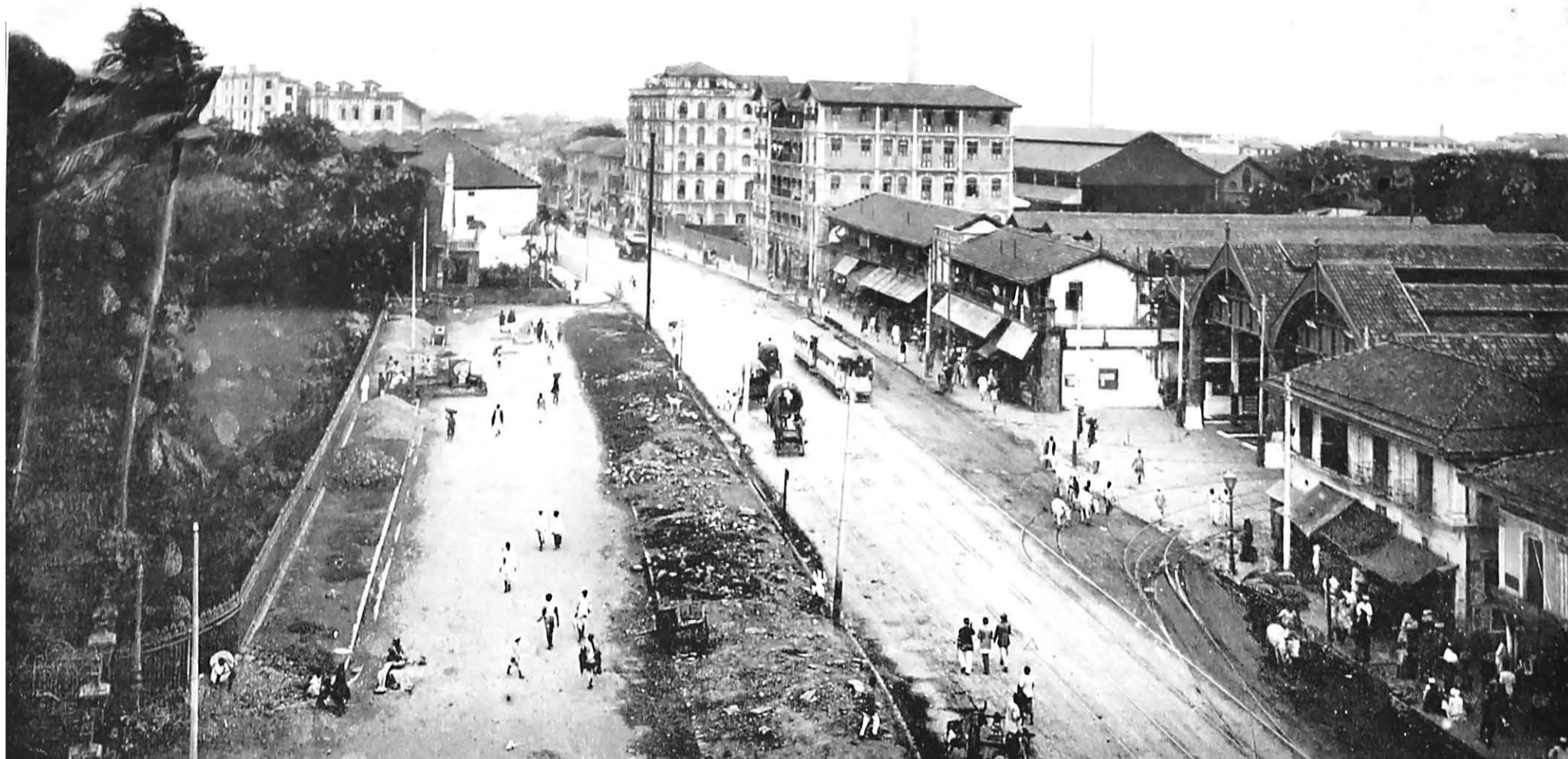
Parel Road and Guzri Bazar South of Victoria Gardens, to be widened to 120 feet.
