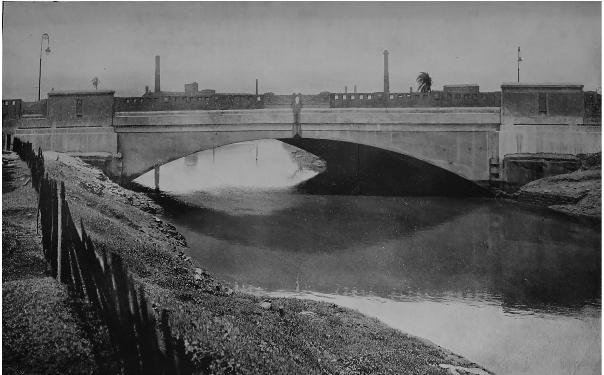
New Reinforced Concrete Bridge at Worli.
