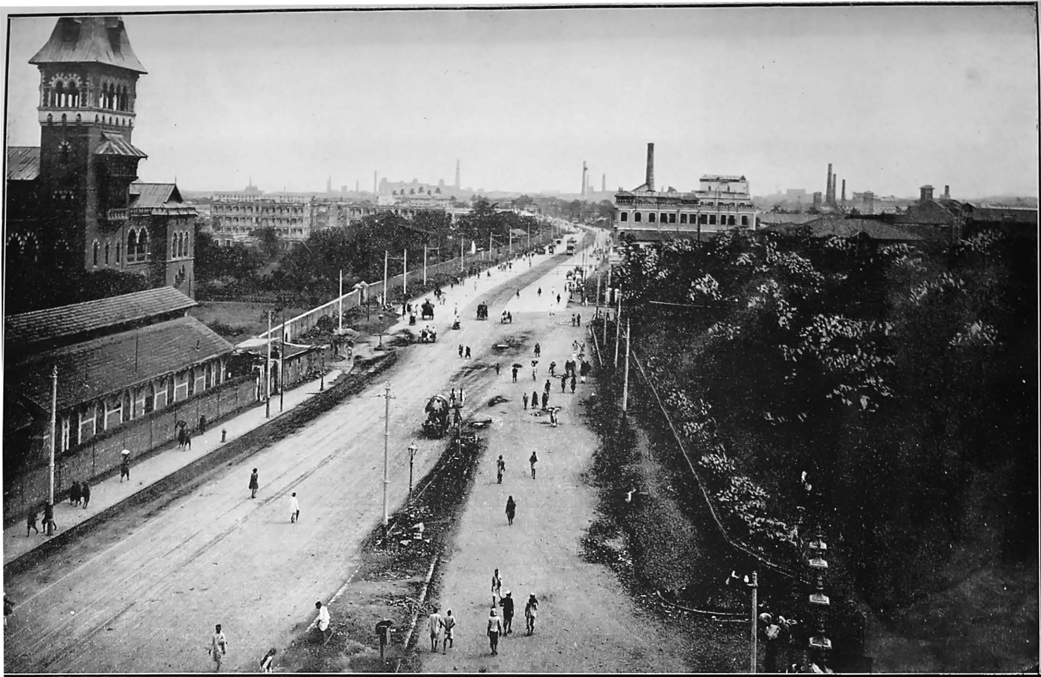
120 Feet Eastern Avenue. Widening of Parel Road, North of Victoria Gardens.
