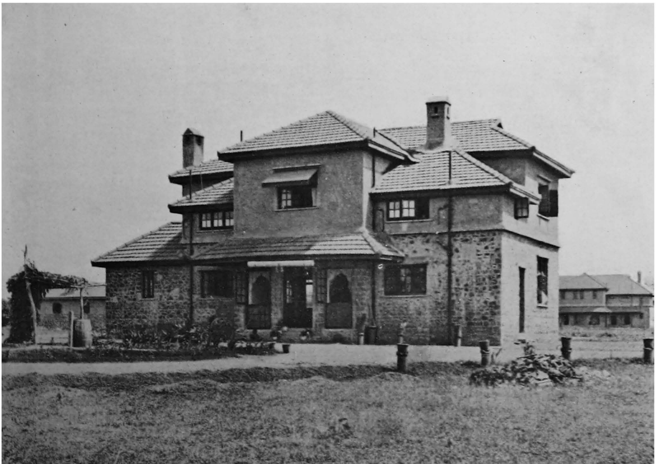
Acetone Factory, Nasik—Works Manager's Bungalow, South view.
