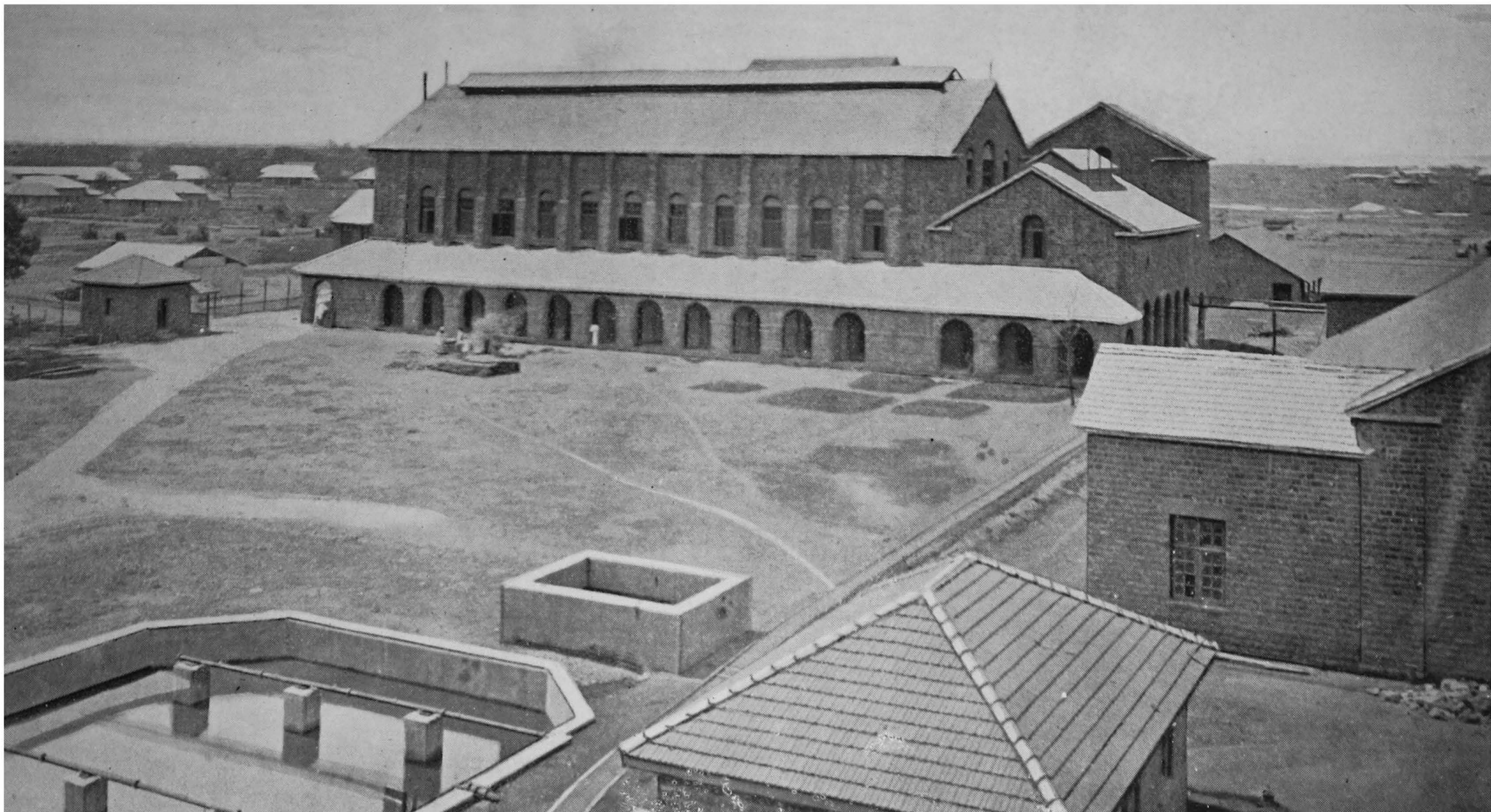
Acetone Factory, Nasik – Vat house and coolie house building.
