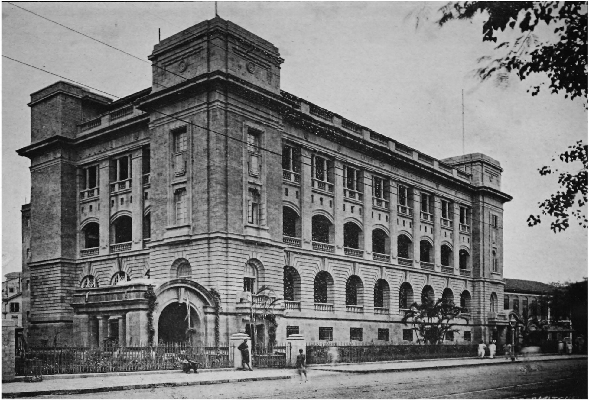
New Small Causes Court, Bombay—South-west view.
