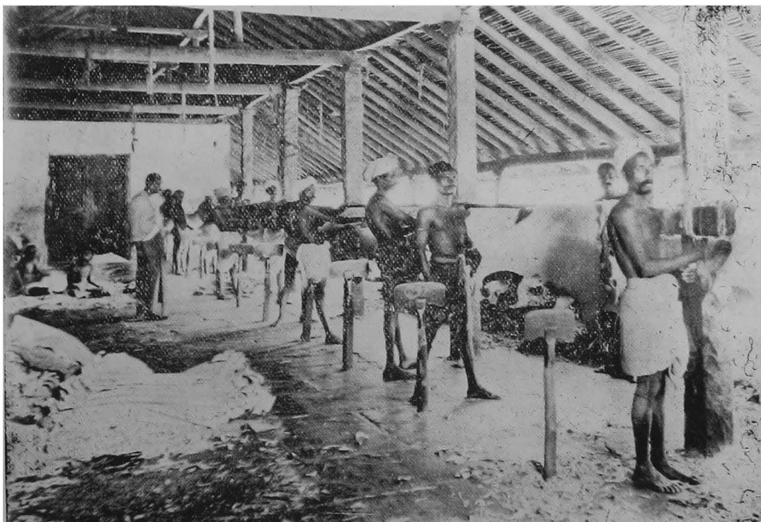
No. L-4.—FLUFFING SKINS ( i.e. , cleaning the flesh side).
