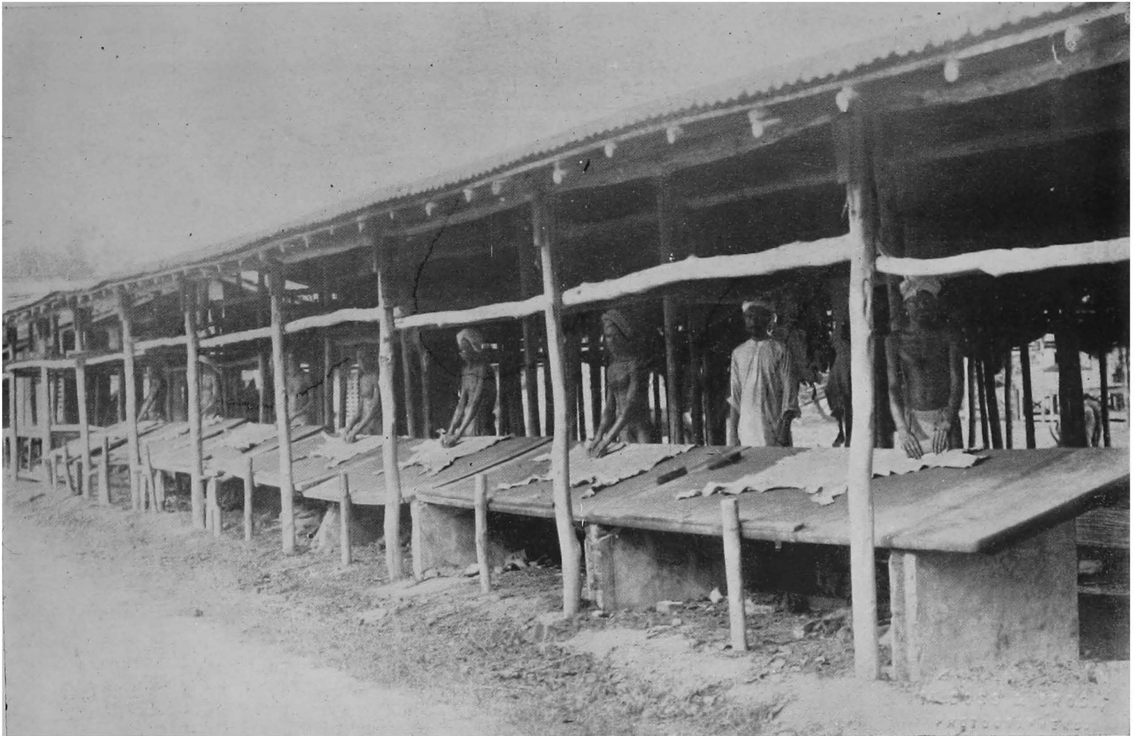
No. L-6.—SETTING OUT HIDES WITH BRASS SLICKERS.
