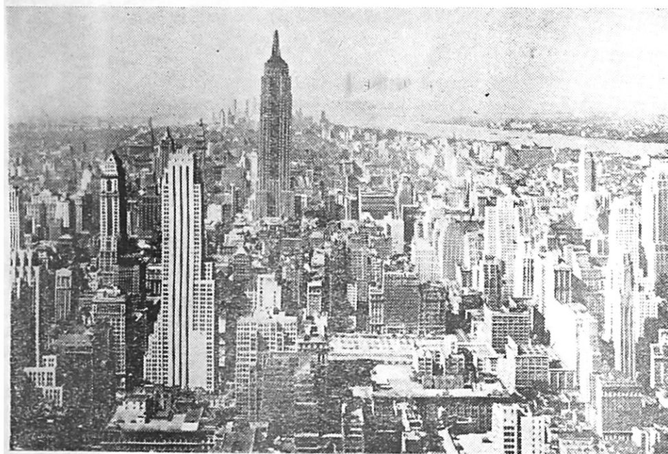
A general view of the Sky-scrapers of New York.
