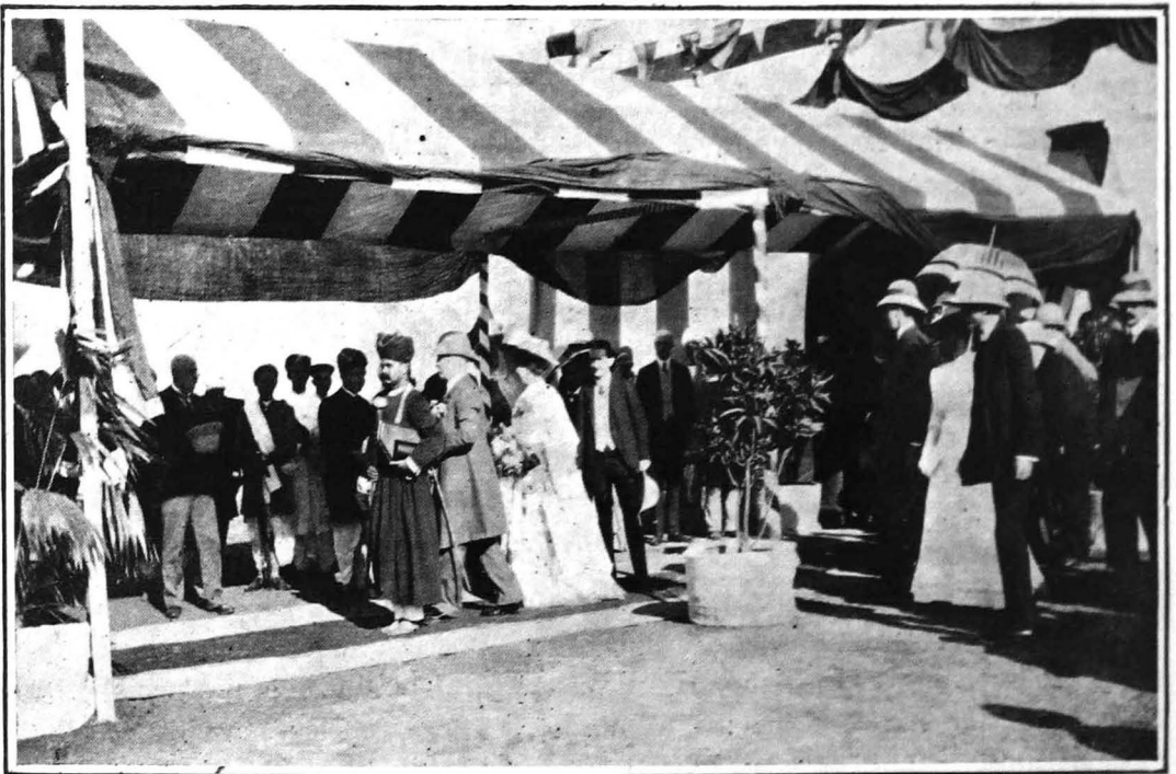
HIS EXCELLENCY PROCEEDING TO LAY THE FOUNDATION STONE.
