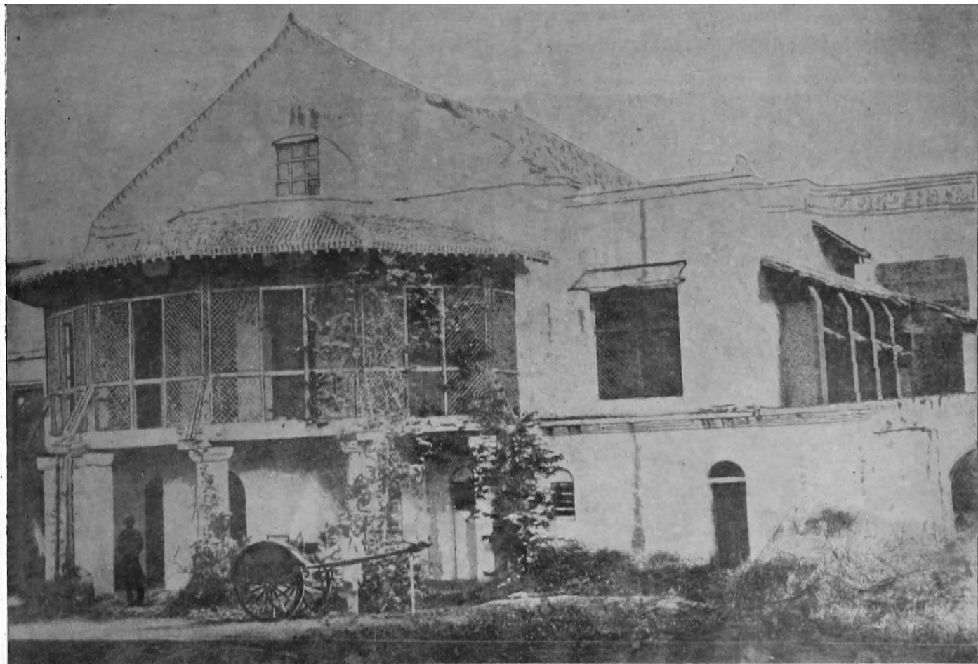
OUTRAM'S BUNGALOW, DHARANGAON.
