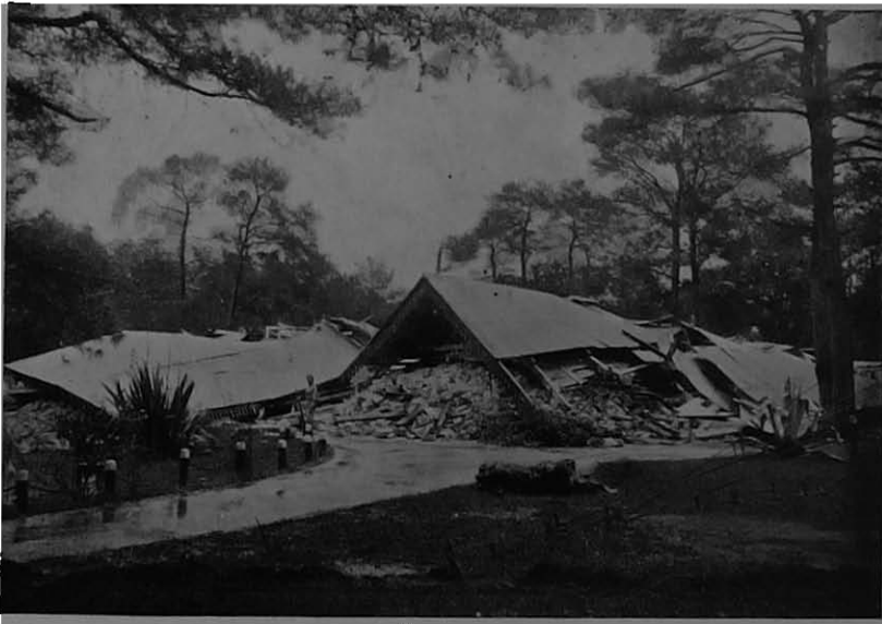
GOVERNMENT HOUSE, SHILLONG, BEFORE AND AFTER THE EARTHQUAKE, 1897.
