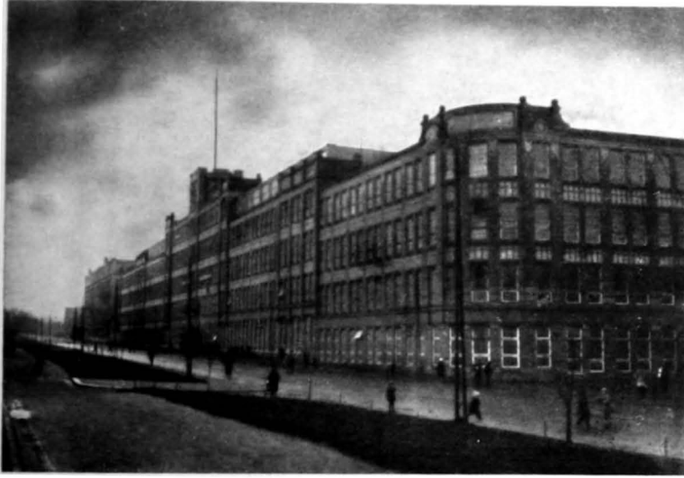
The Swedish Ball-Bearing Factory at Göteborg (SKF). In this block of buildings there are manufactured every day 15,000 ball- and roller-bearings.
