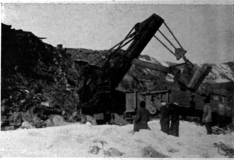
Surface Quarrying at K urunavaara Loading ore-trucks by means of electric ore-grabs
