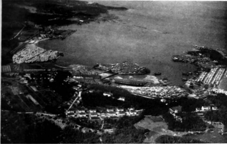
Skutskär Sawmill at the mouth of the River Dalälven (Stora Kopparbergs Bergslags A.-B.).
