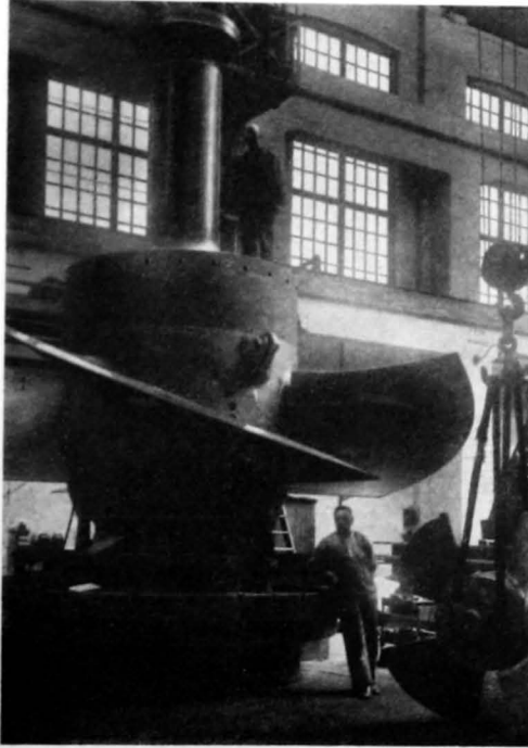
Water-turbine wheel in course of construction (Karlstads Mek. Verkstads A.-B.).
