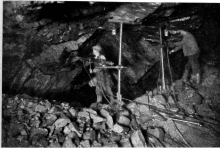
Underground Mining at Striberg Shrinkage stoping with pneumatic rock-drills
