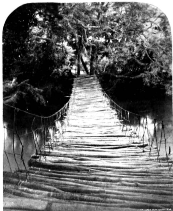
NATIVE BRIDGE OVER THE LUFU.
