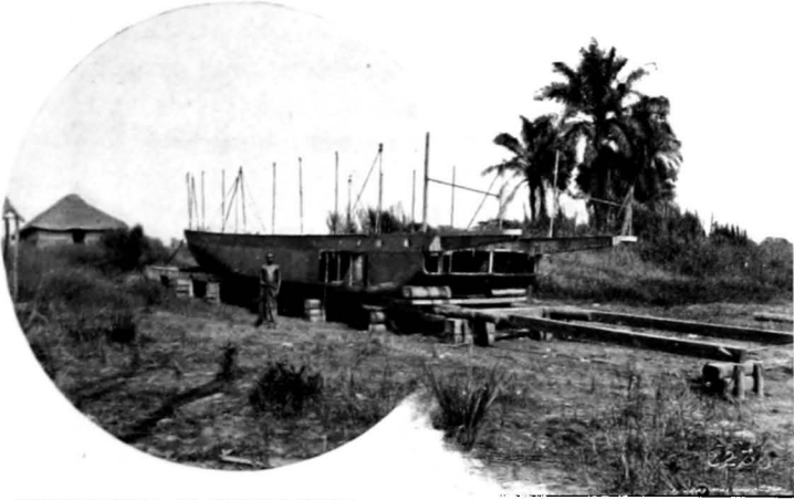
SHIPBUILDING AT LEOPOLDVILLE.
