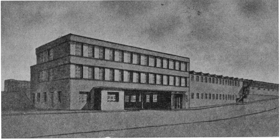
The Kammgarn factory in construction
