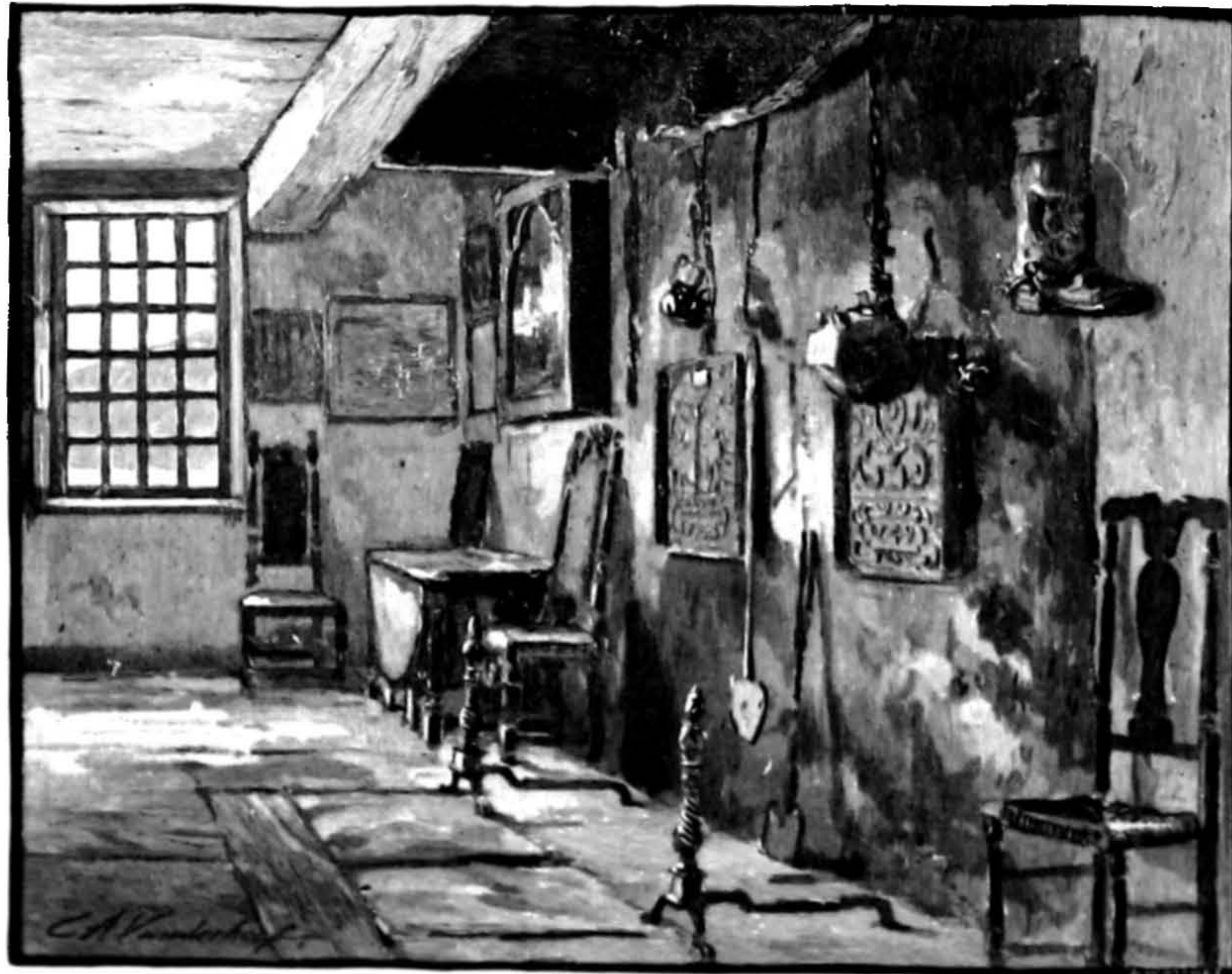
INTERIOR OF WASHINGTON'S HEADQUARTERS, NEWBURG
