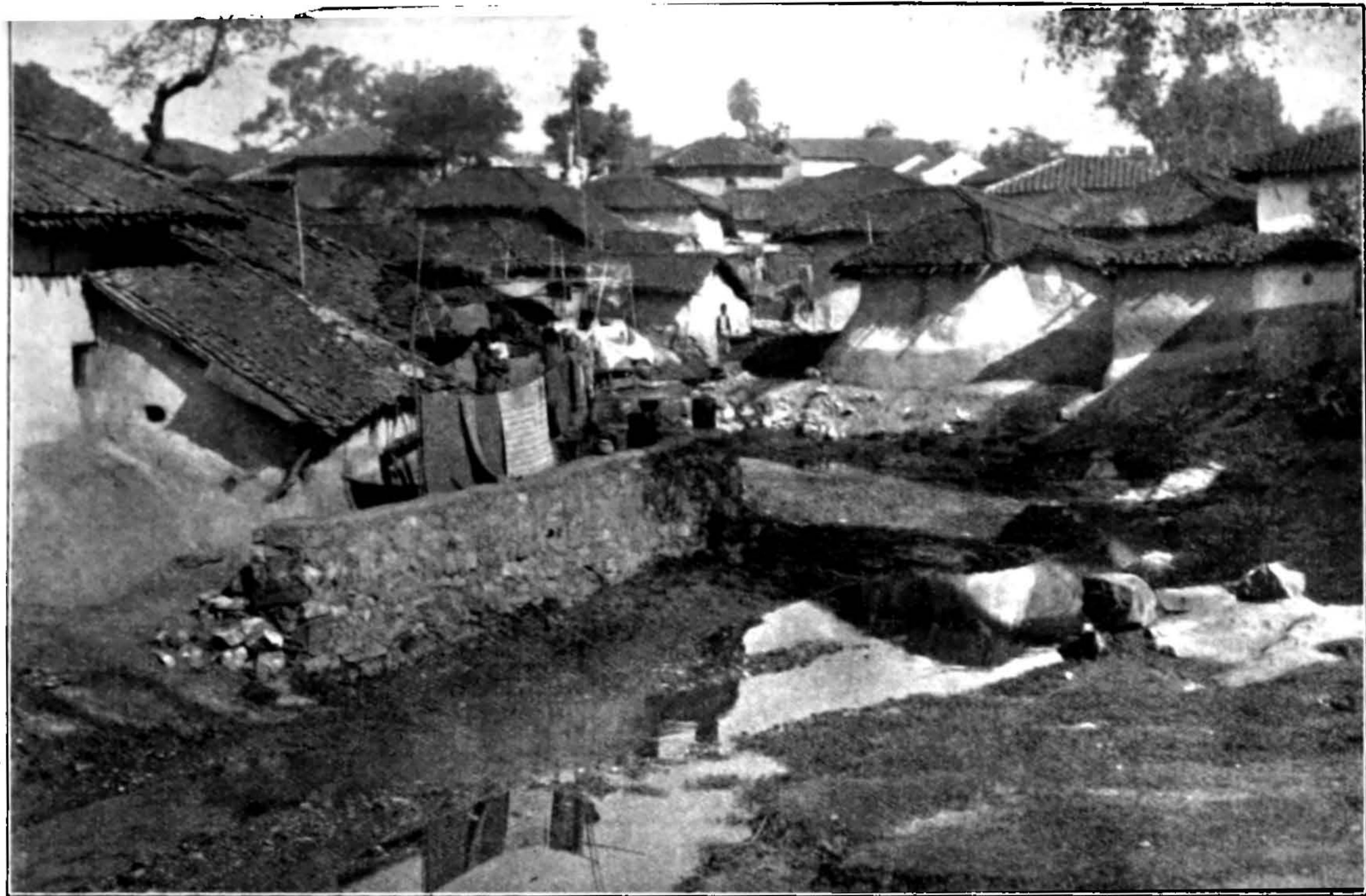
A TEXTILE WORKERS' VILLAGE. SHOWING OPEN DRAIN.
