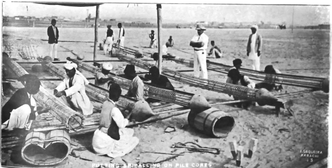
10—New Customs House, Karachi—Putting spiralling on pile cores.
