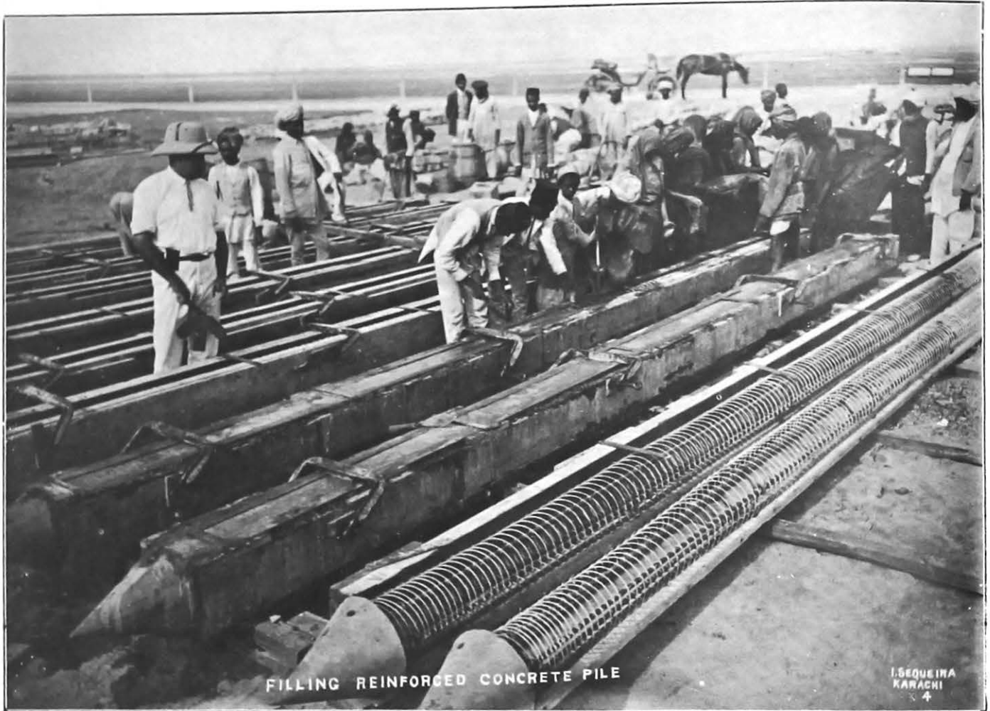
11—New Customs House, Karachi—Filling reinforced concrete piles.
