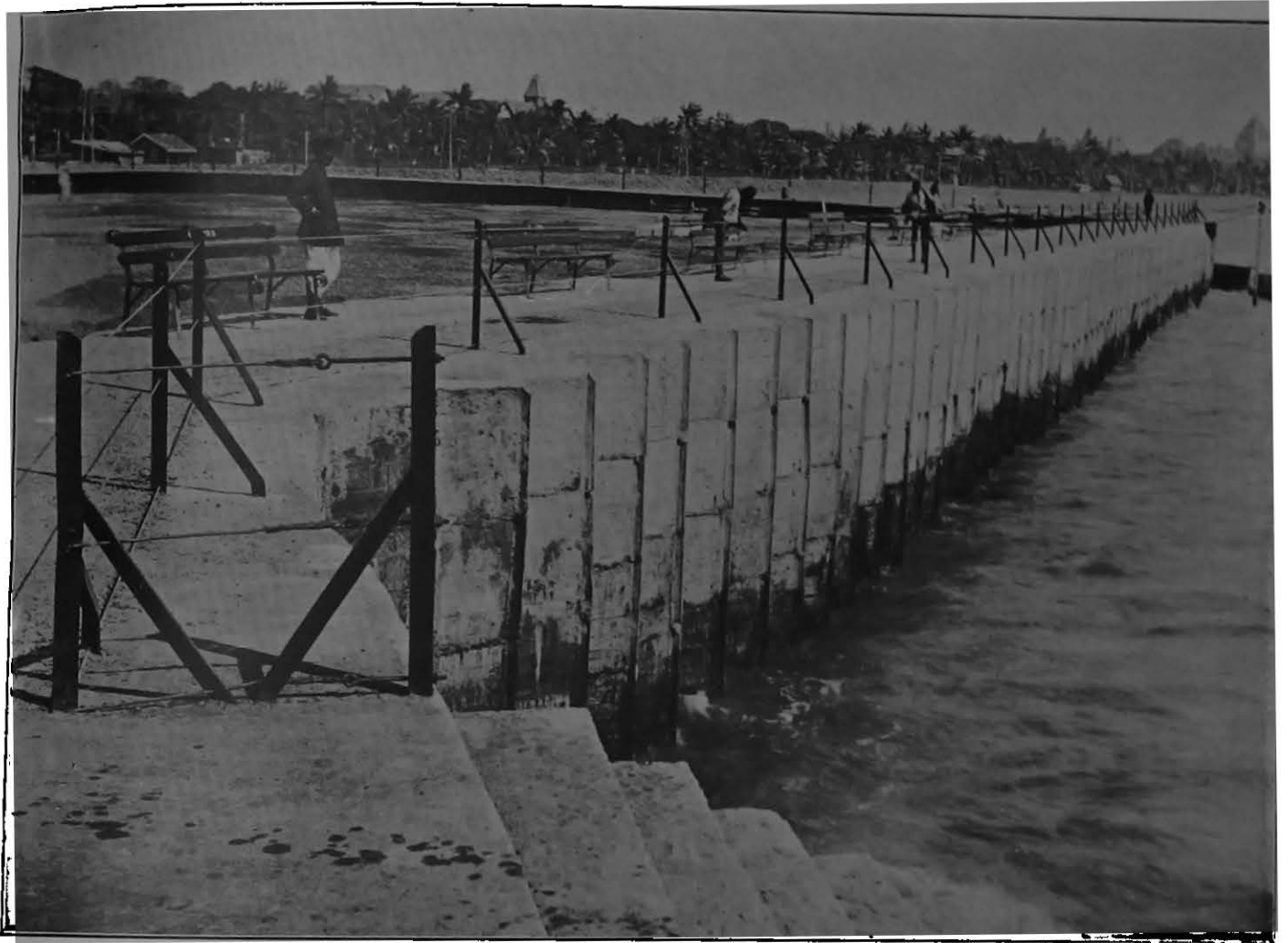
5—Kennedy Sea Face, Bombay—Vibrocel Wall. 13th April 1915.
