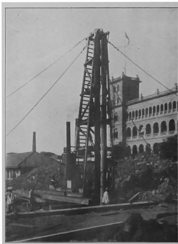
BOMBAY CUSTOMS HOUSE. REINFORCED CONCRETE PILE DRIVING.
