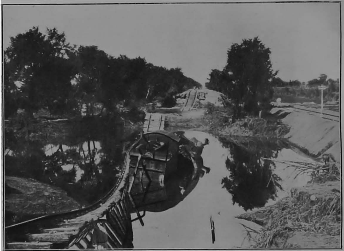
Engine in breach near Lhaksar, Oudh and Rohilkhand Railway, during the floods.
