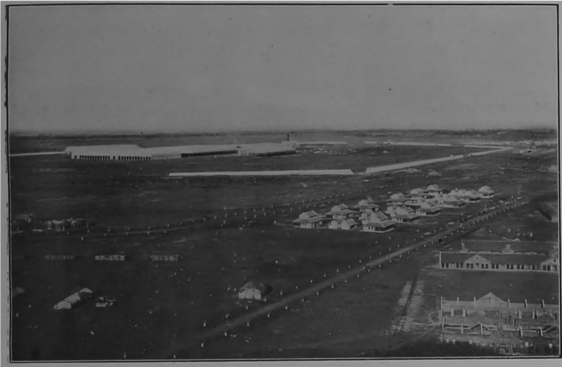
Bird's-eye view of Workshops under Construction.
