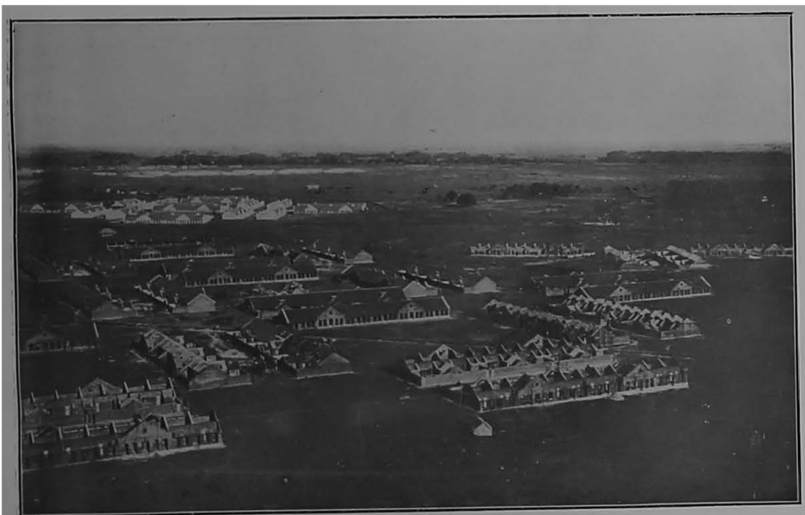
Bird's-eye view of Staff quarters under Construction.
