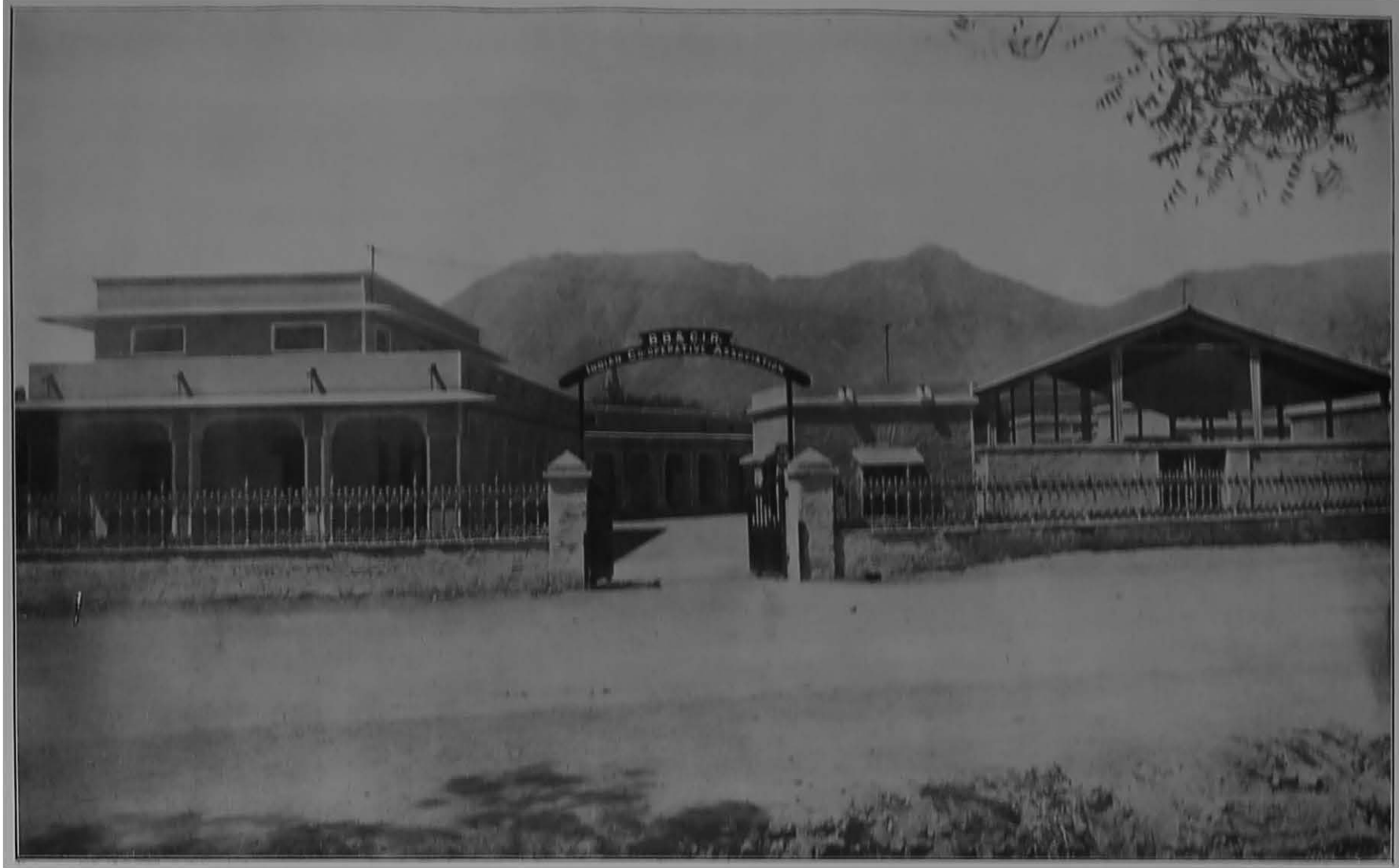
Bombay, Baroda and Central India Railway Indian Co-operative Association building in Ajmer.
