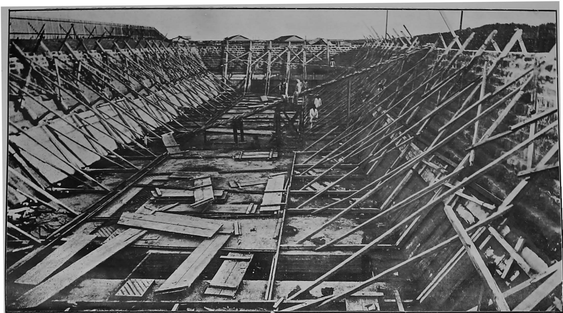
Concrete Lined Tank for Liquid Fuel at Karachi—North Western Railway.
