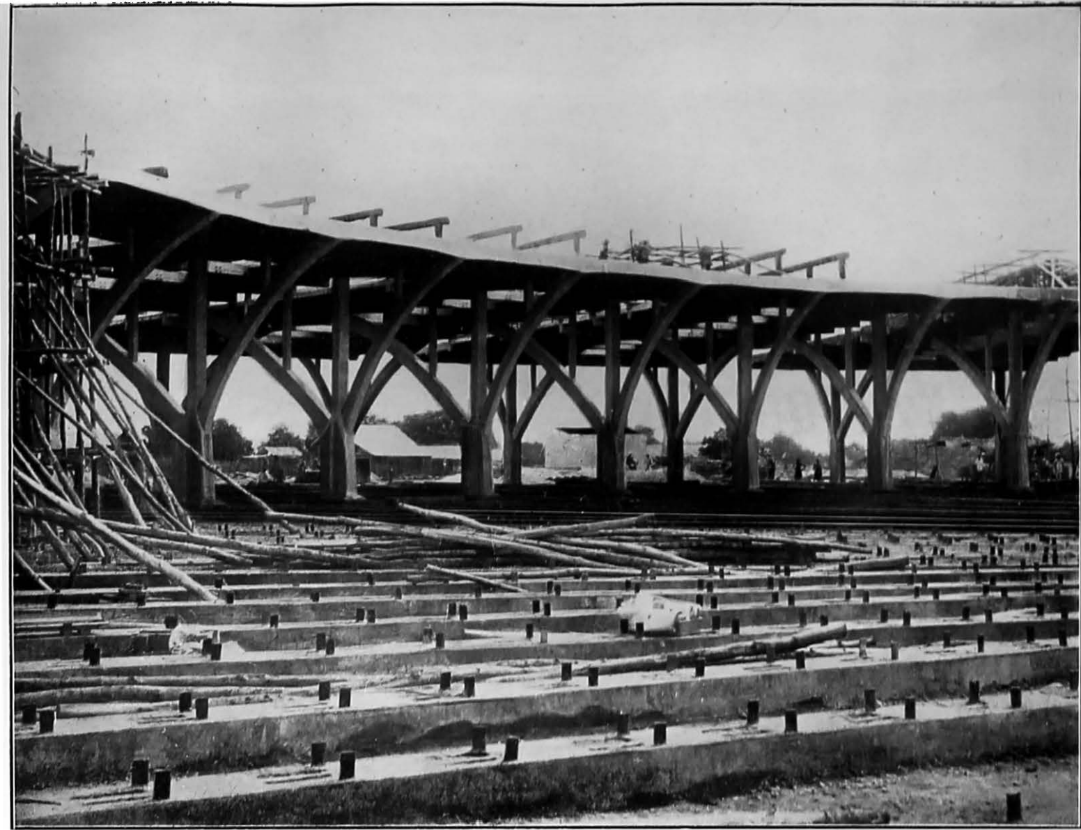
Reinforced concrete Engine Round House under construction at Bitragunta.
