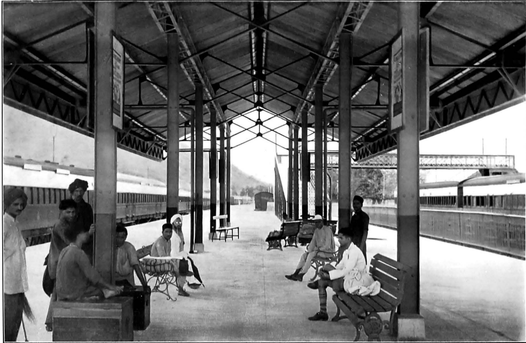
Newly constructed platform shed at Hardwar station.
