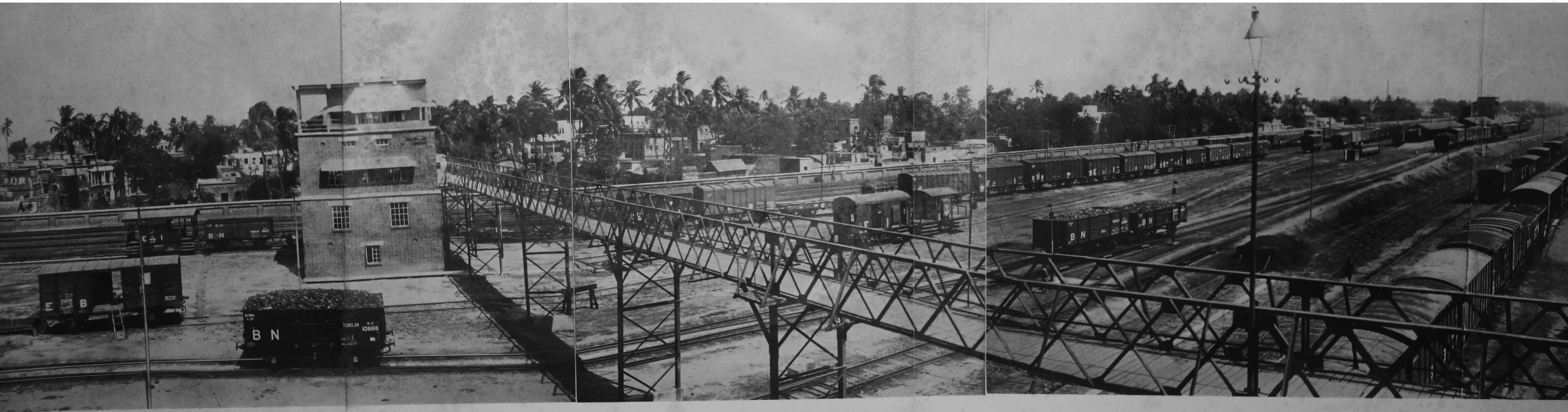
Panoramic view of the hump yard at Naihati.
