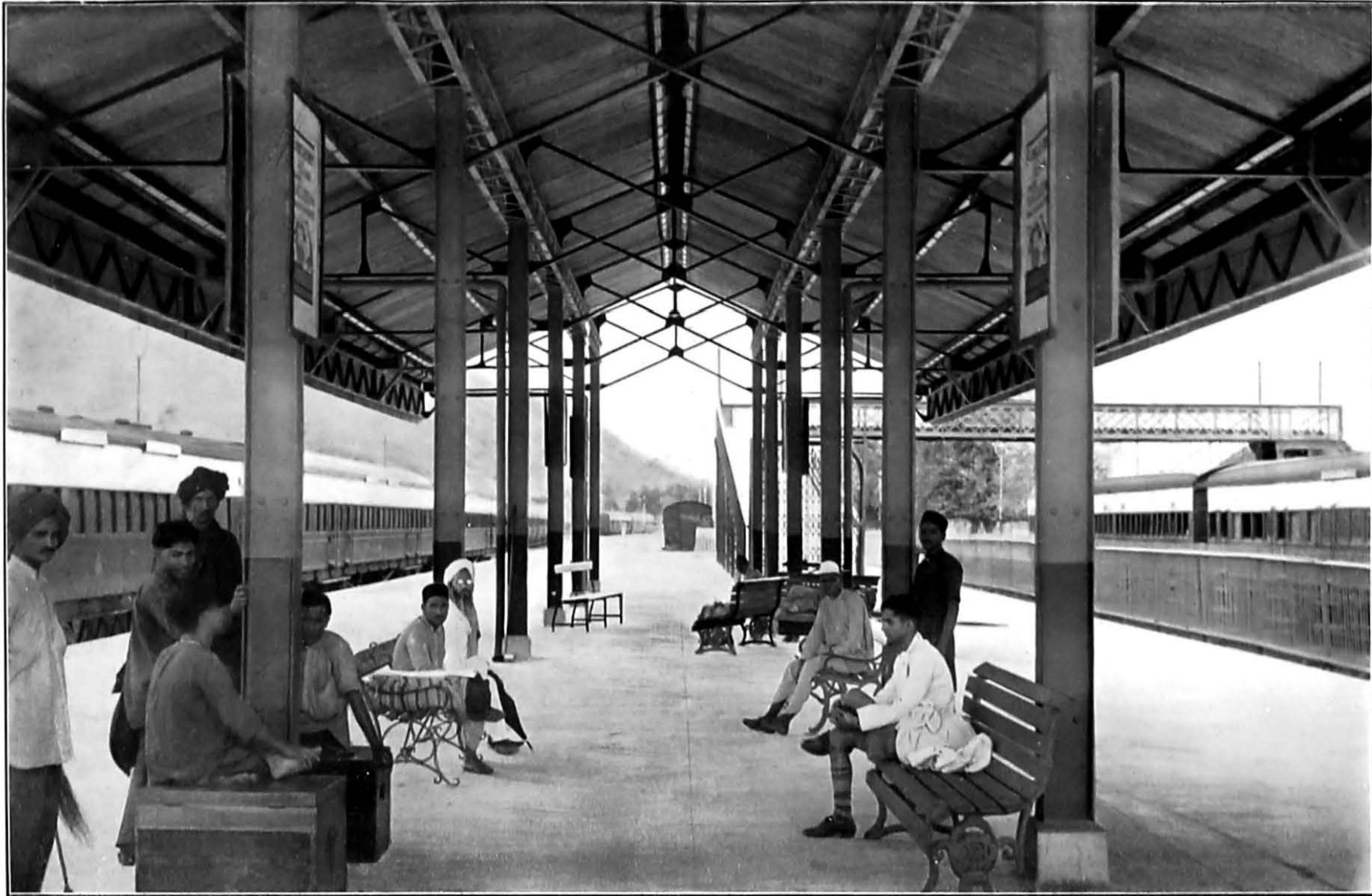
Newly constructed platform shed at Hardwar station.
