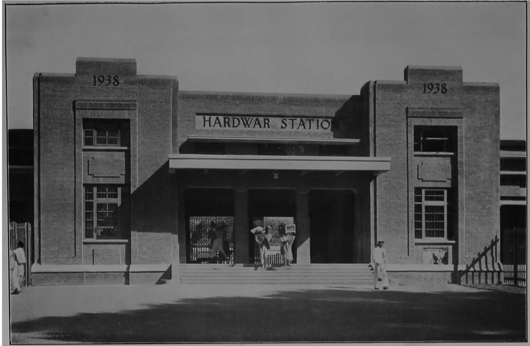
Facade of the new station at Hardwar.
