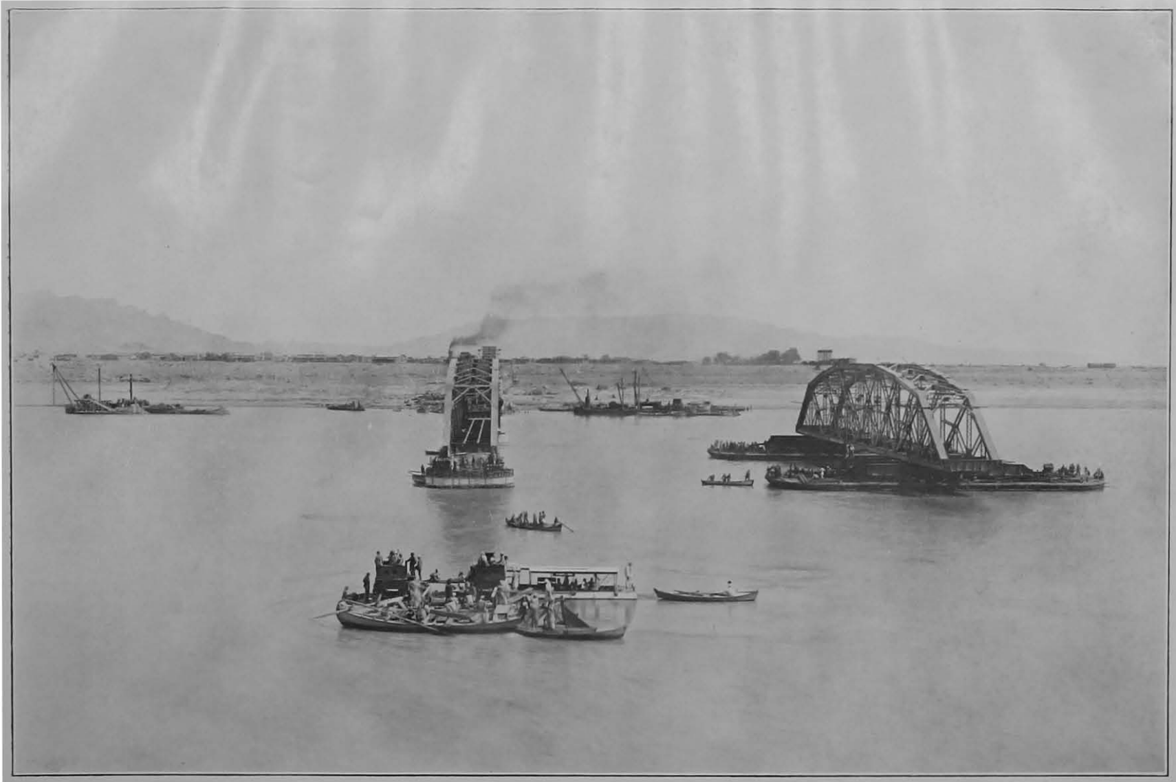
Kalabagh Bridge, Floating Span No. 6 in position.
