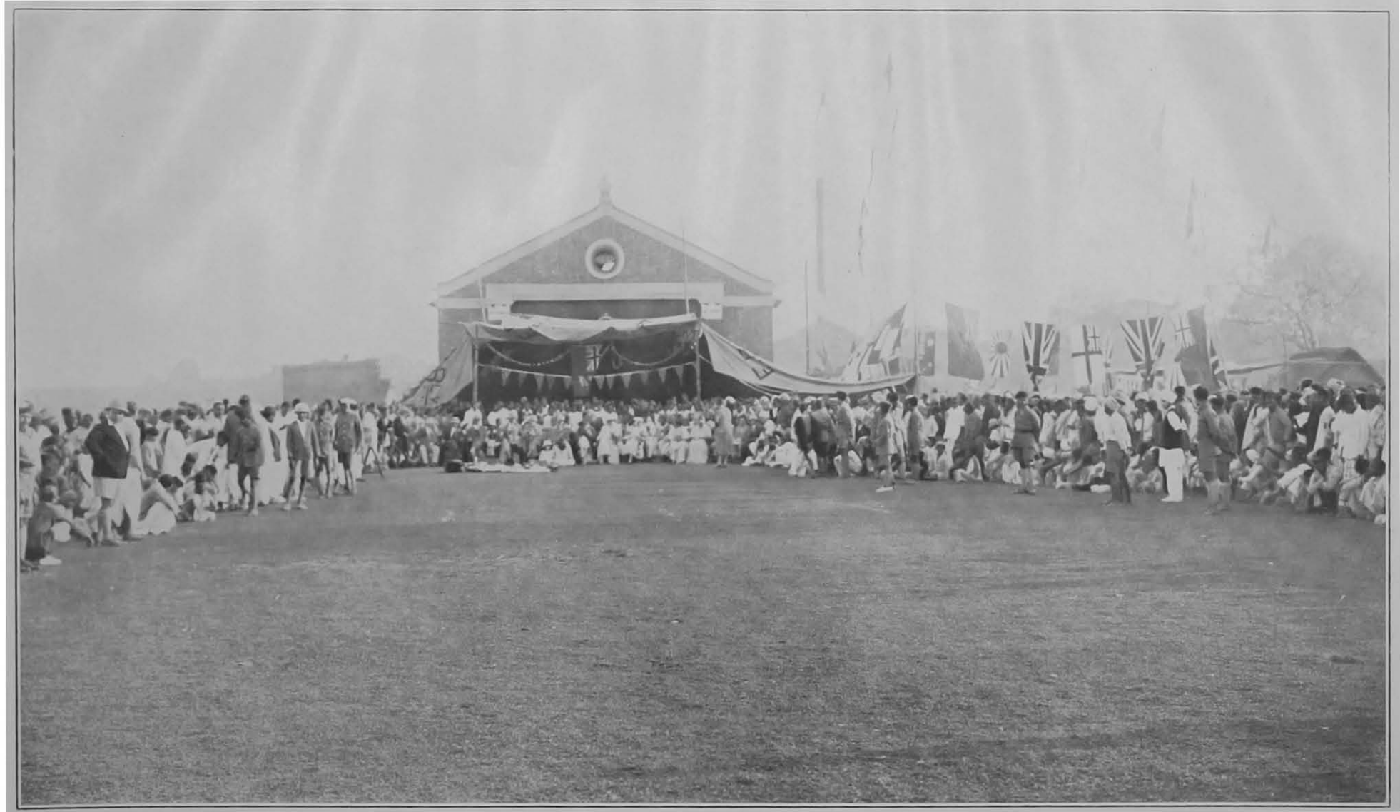
Workmen's Institute, Saidpur.
