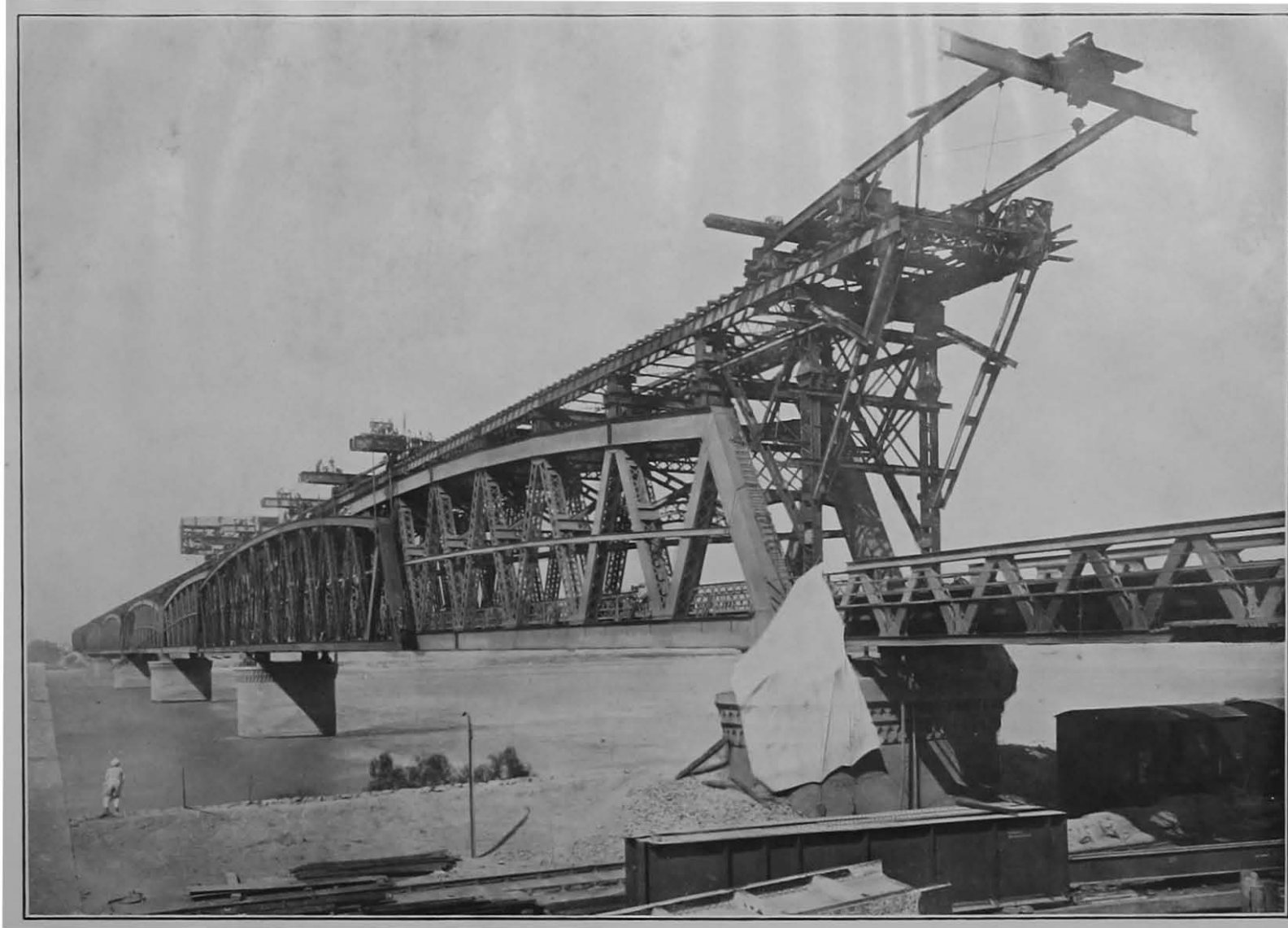
Strengthening Indus Bridge at Kotri.
