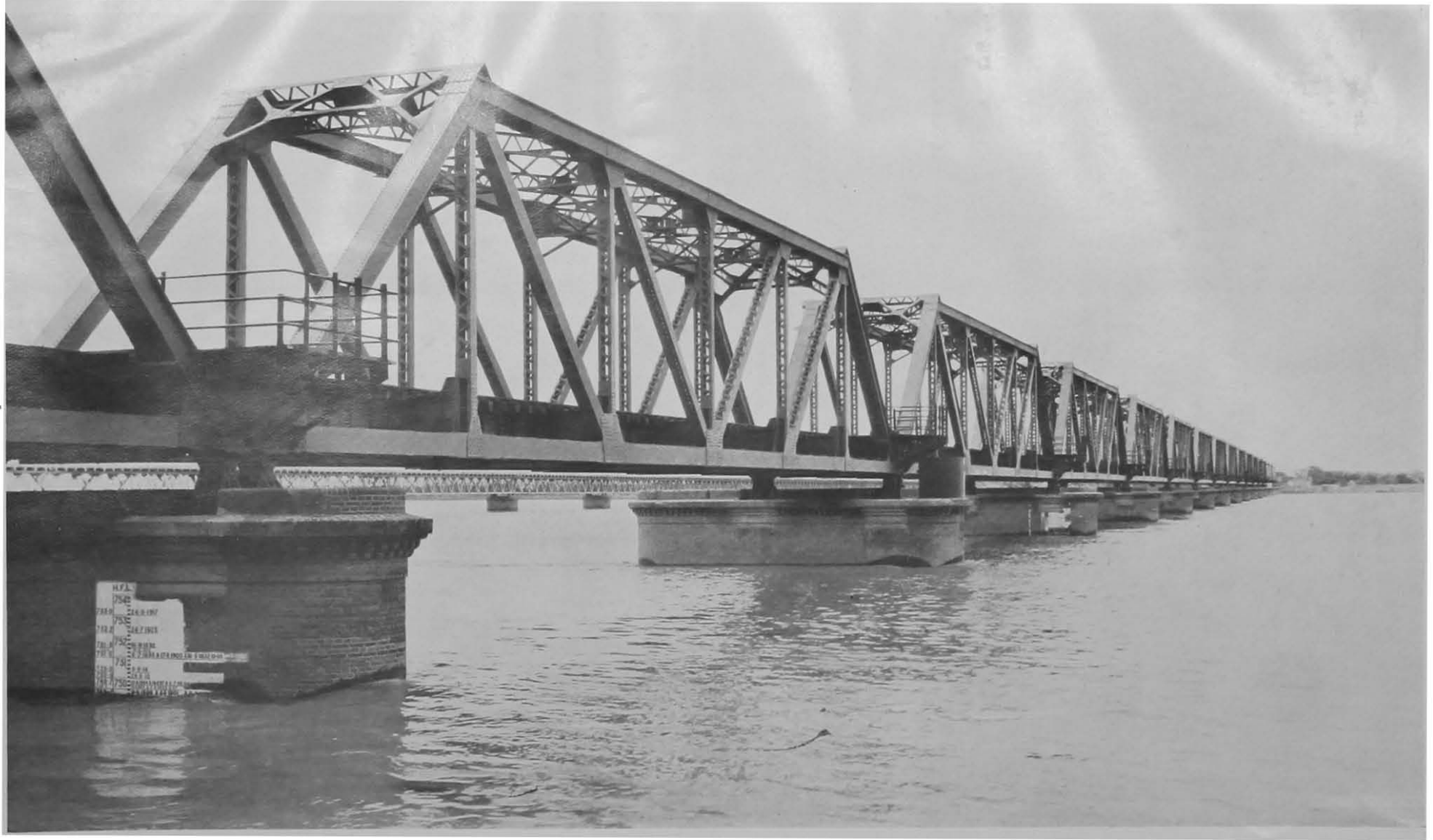
VIEW OF COMPLETED BRIDGE.
