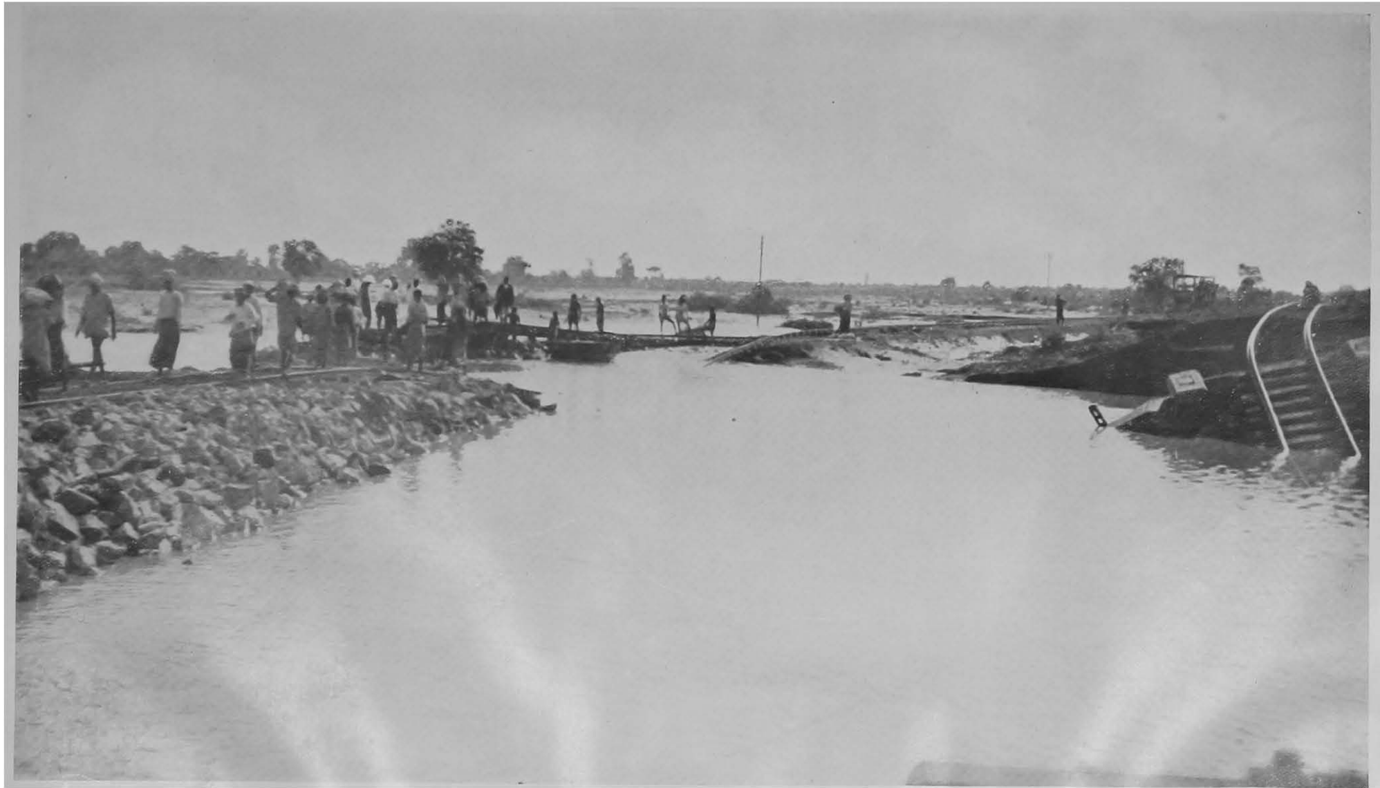
BREACH AT BRIDGE 192, MILE 335-1.
