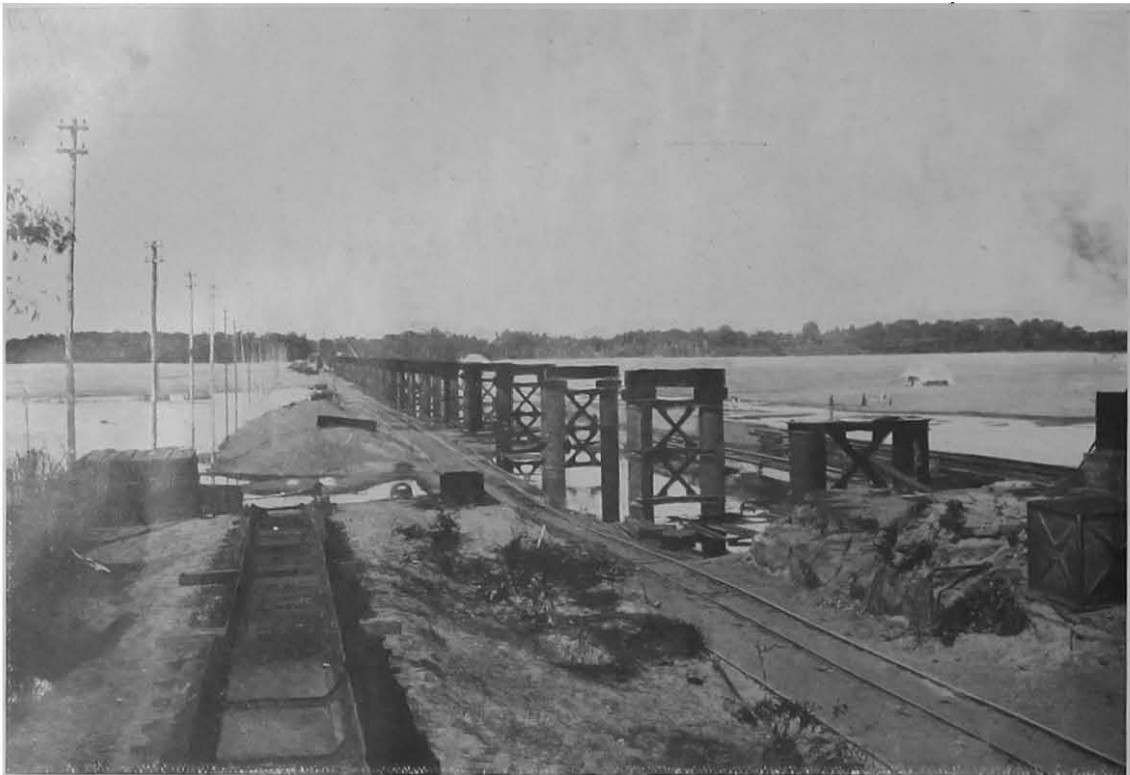
SHOWING OPERATIONS AT THE 39TH SPAN.
