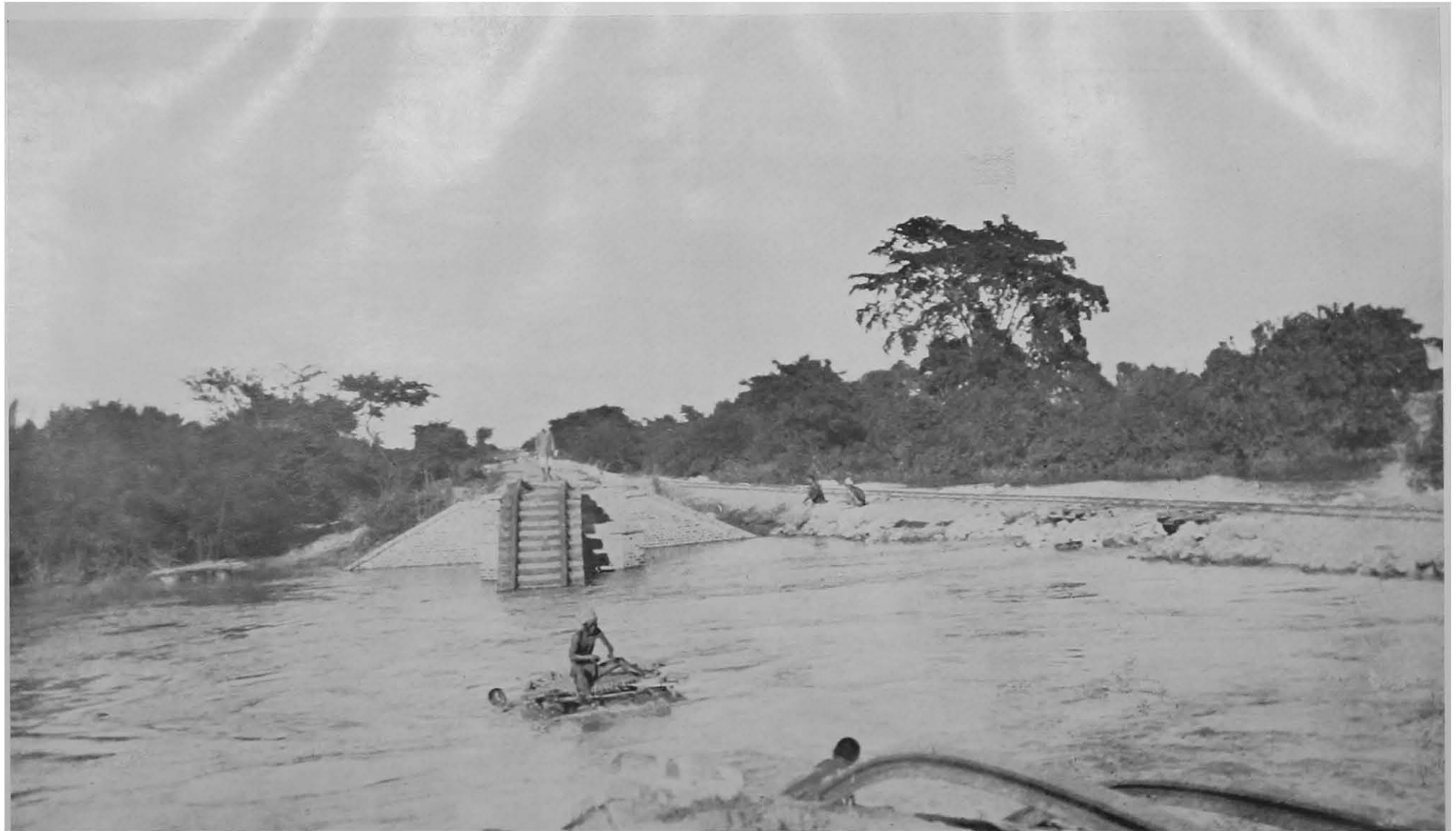
BREACH AT BRIDGE 192, MILE 335-1.
