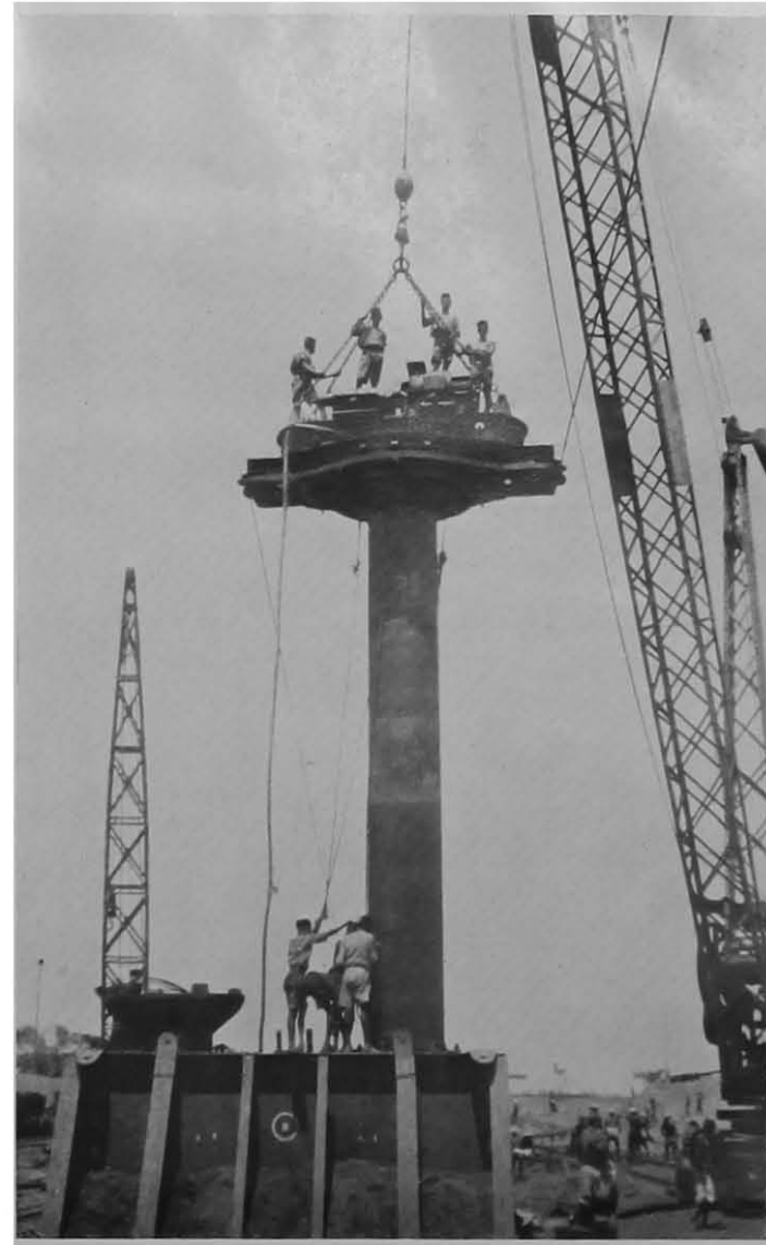
VIEWS SHEWING SCREWING OPERATIONS OF CYLINDERS.
