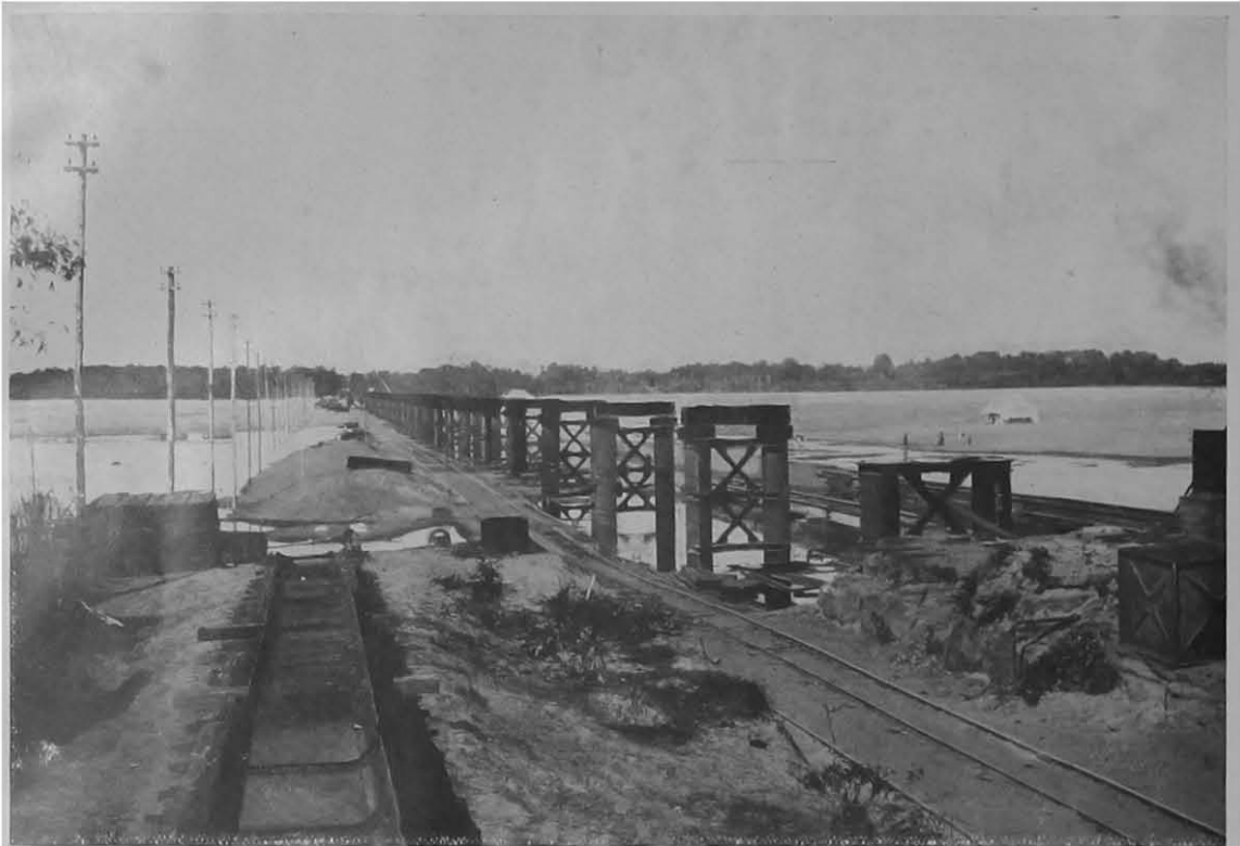
SHOWING OPERATIONS AT THE 39TH SPAN.
