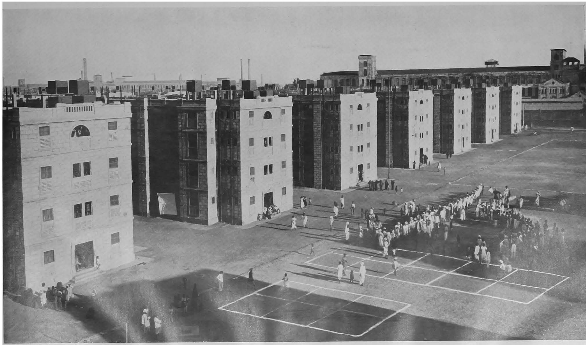
GENERAL VIEW SHEWING CHAWLS OCCUPIED BY BOMBAY, BARODA & CENTRAL INDIA RAILWAY WORKSHOPS EMPLOYEES AT WORLI (BOMBAY).
