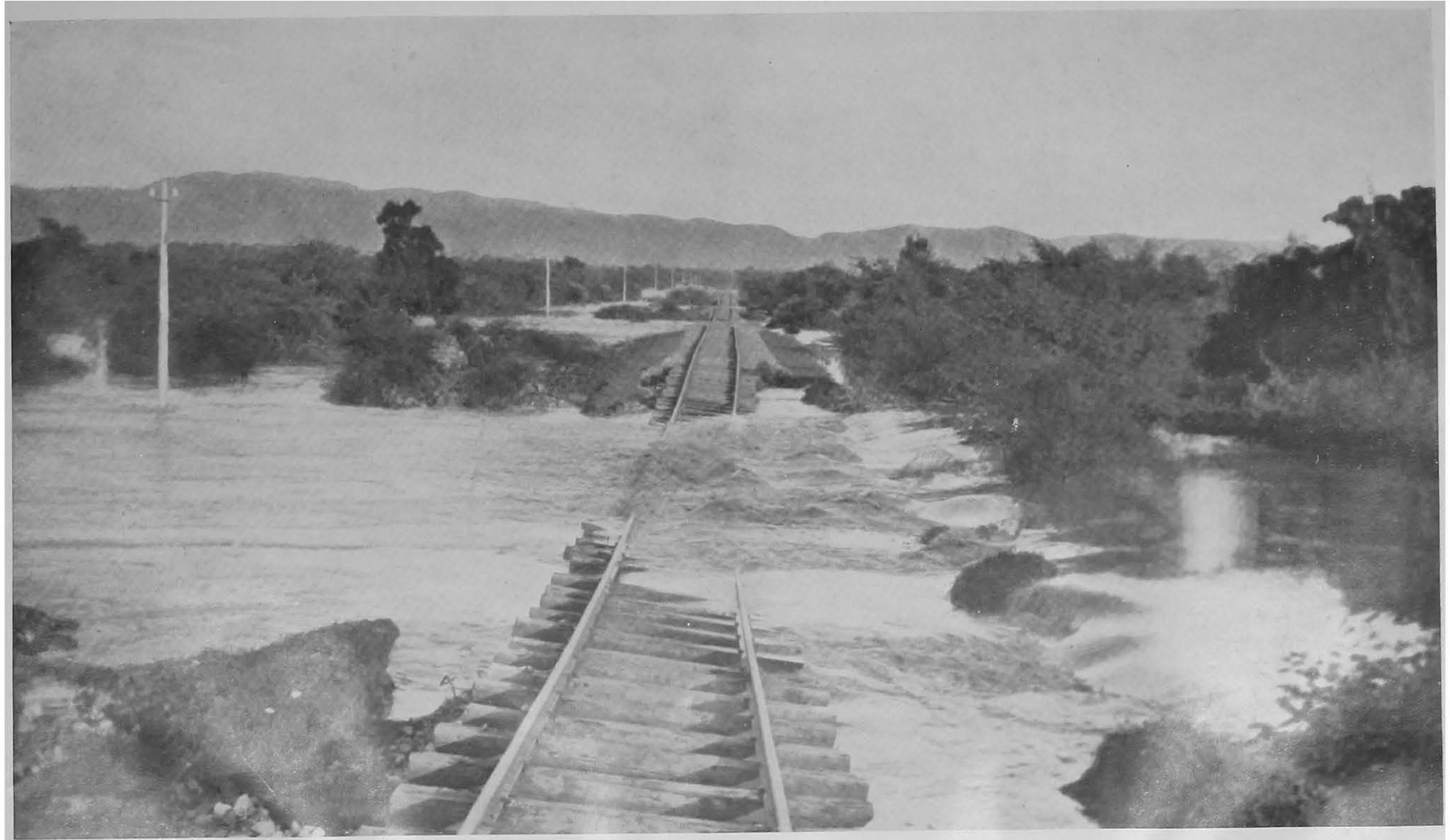
FLOODS NEAR HLAINGDET (SOUTHERN SHAN STATES RAILWAY).
