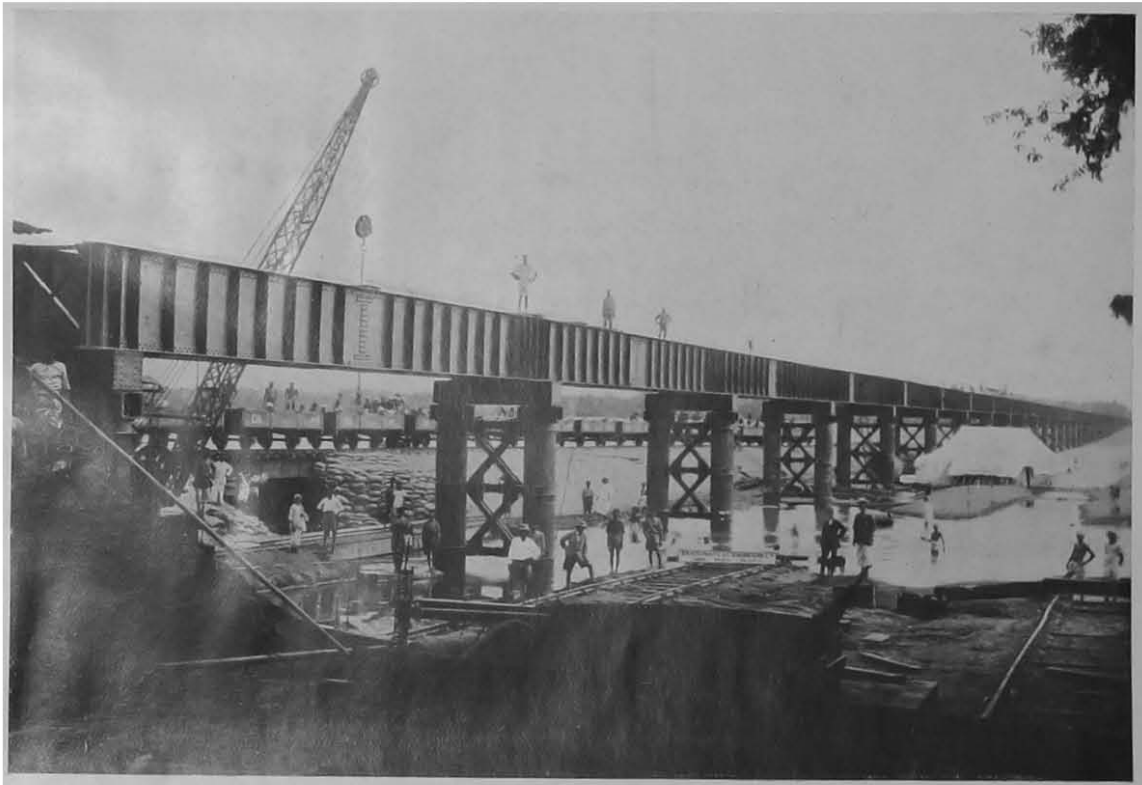
VIEW OF BRIDGE COMPLETE.
