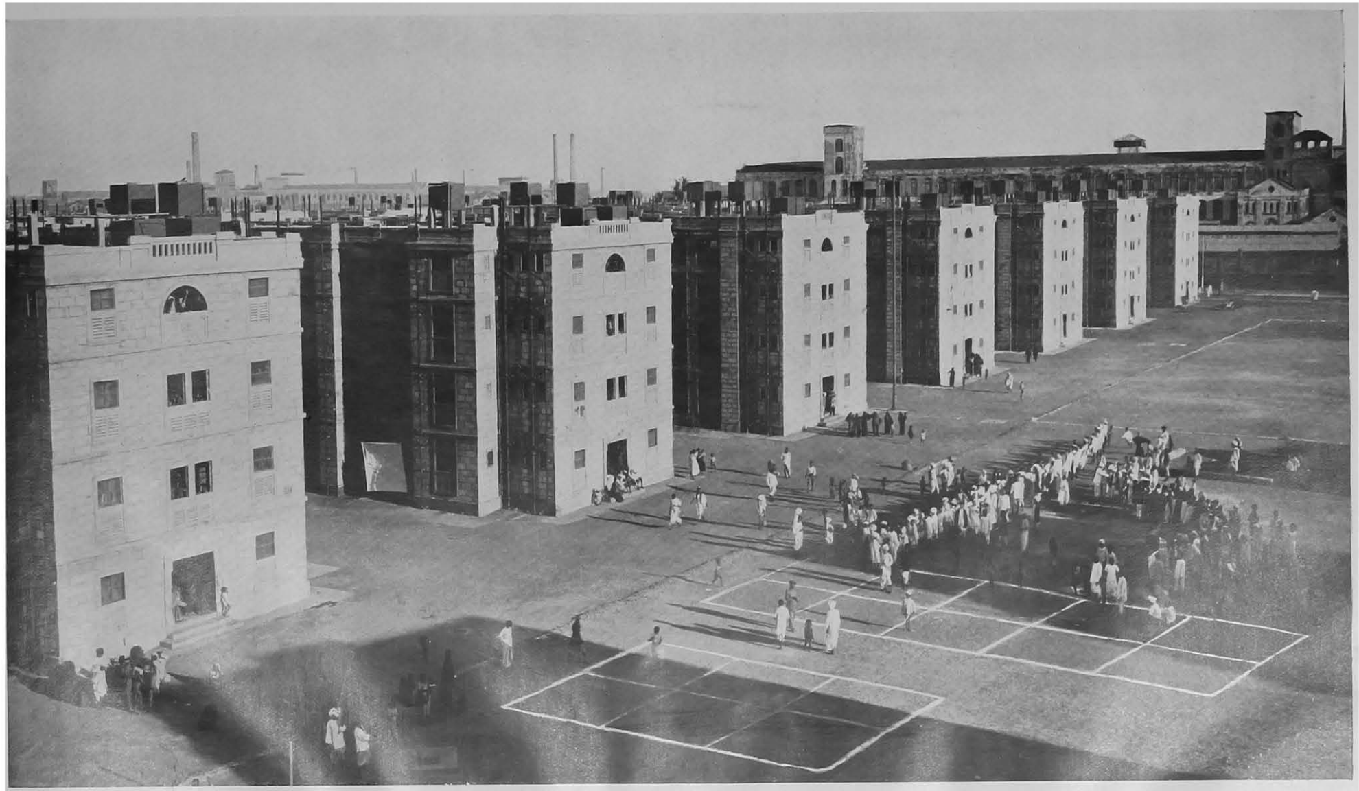
GENERAL VIEW SHEWING CHAWLS OCCUPIED BY BOMBAY, BARODA & CENTRAL INDIA RAILWAY WORKSHOPS EMPLOYEES AT WORLI (BOMBAY).
