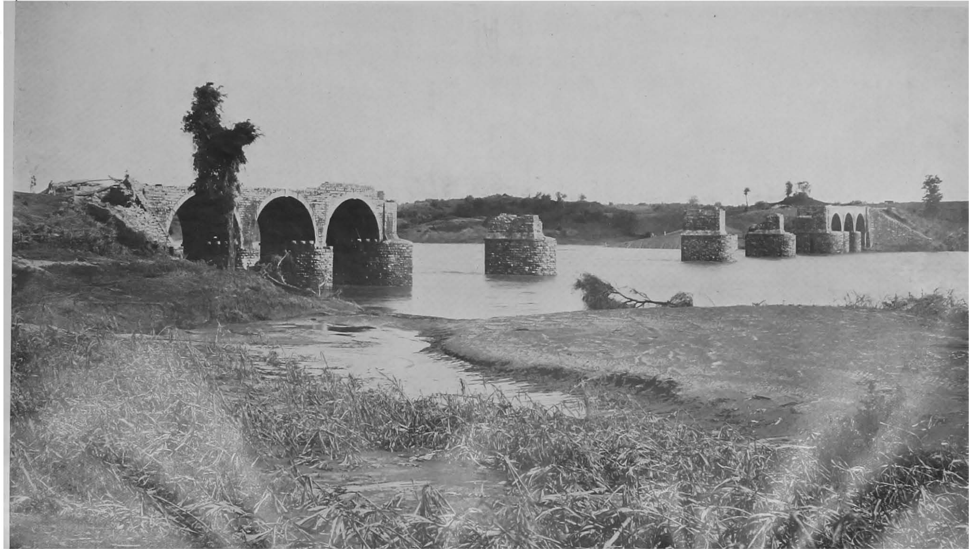
PIERS LEFT STANDING AFTER THE FLOODS HAD SUBSIDED.
