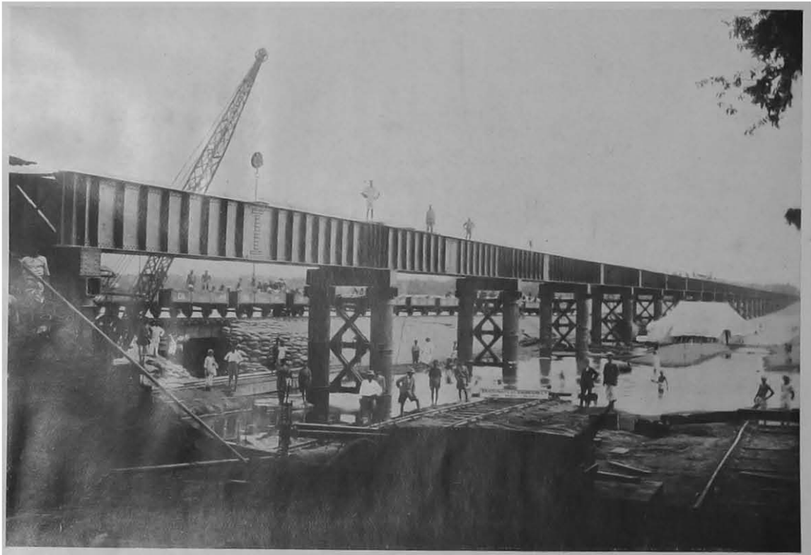
VIEW OF BRIDGE COMPLETE.
