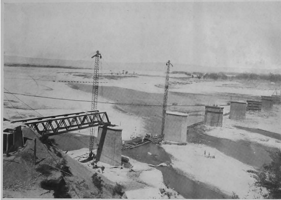
VIEW SHEWING GIRDER ERECTION IN PROGRESS AT GAJ.BRIDGE.
