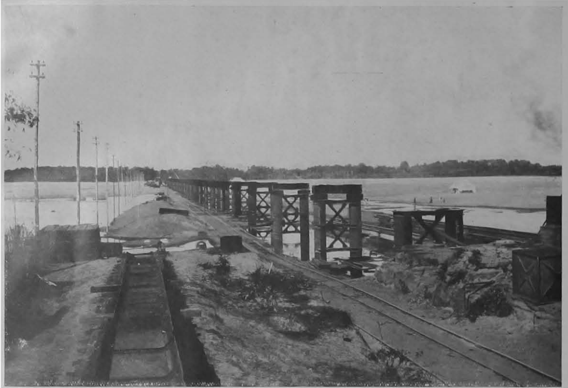
SHOWING OPERATIONS AT THE 39TH SPAN.
