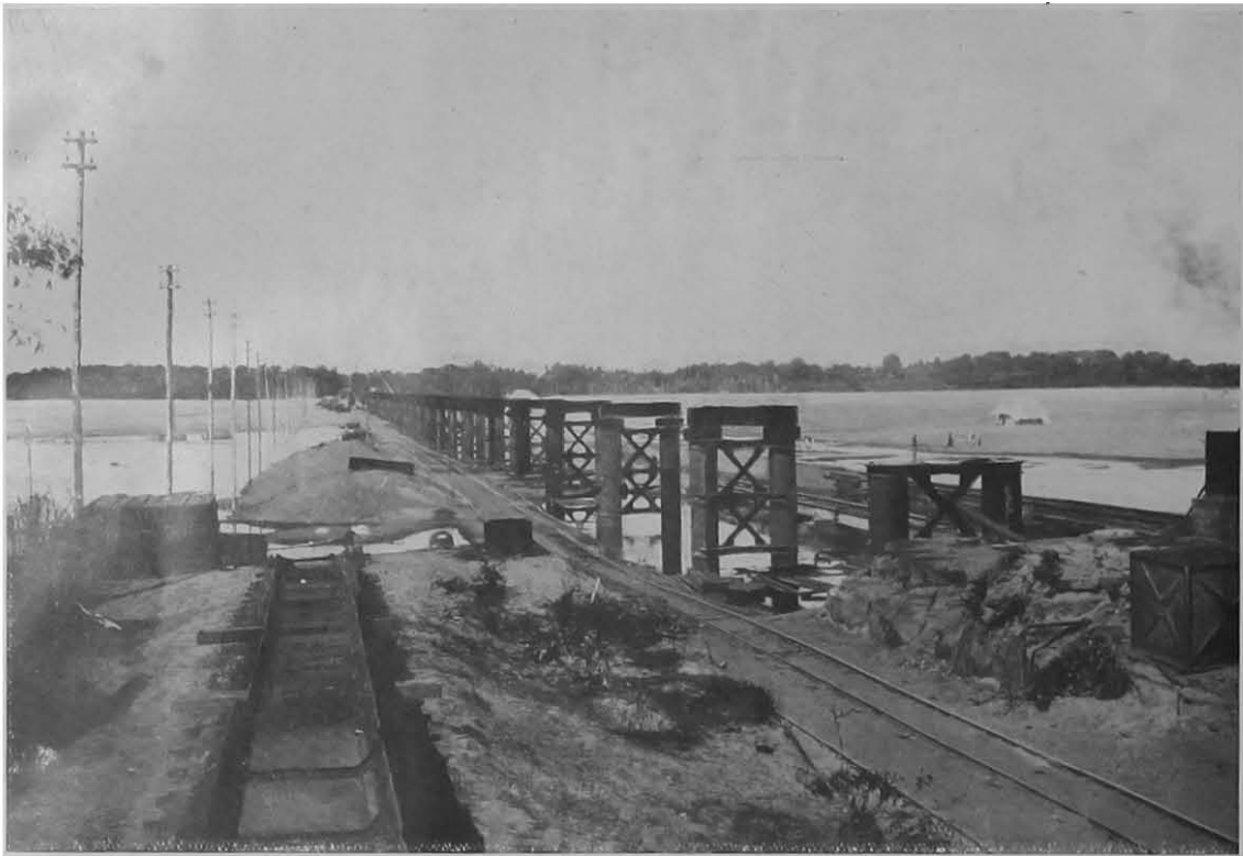
SHOWING OPERATIONS AT THE 39TH SPAN.
