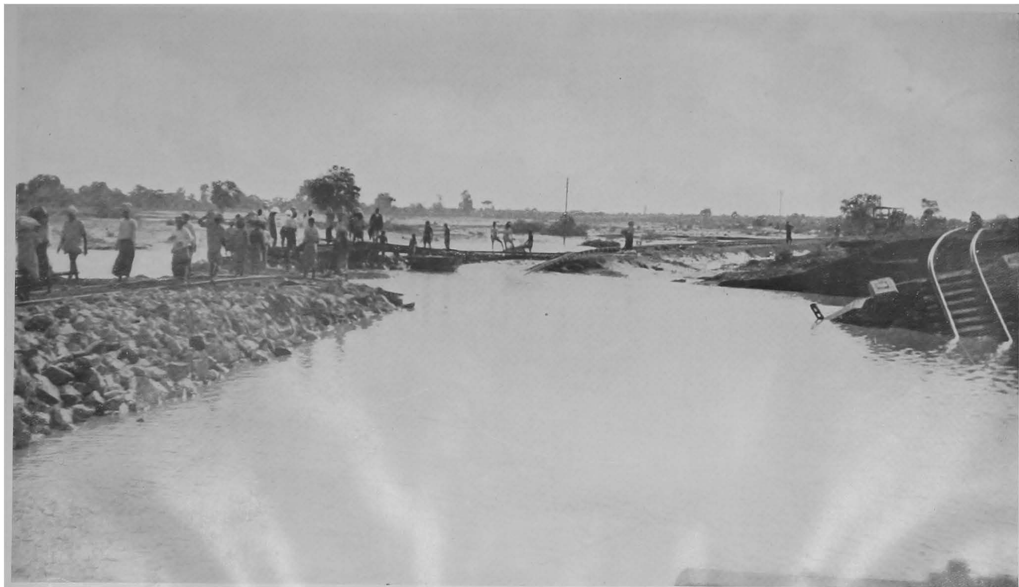
BREACH AT BRIDGE 192, MILE 335-1.
