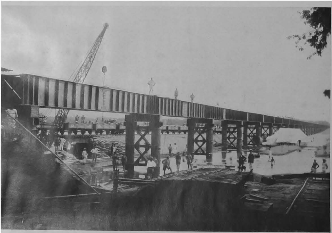
VIEW OF BRIDGE COMPLETE.
