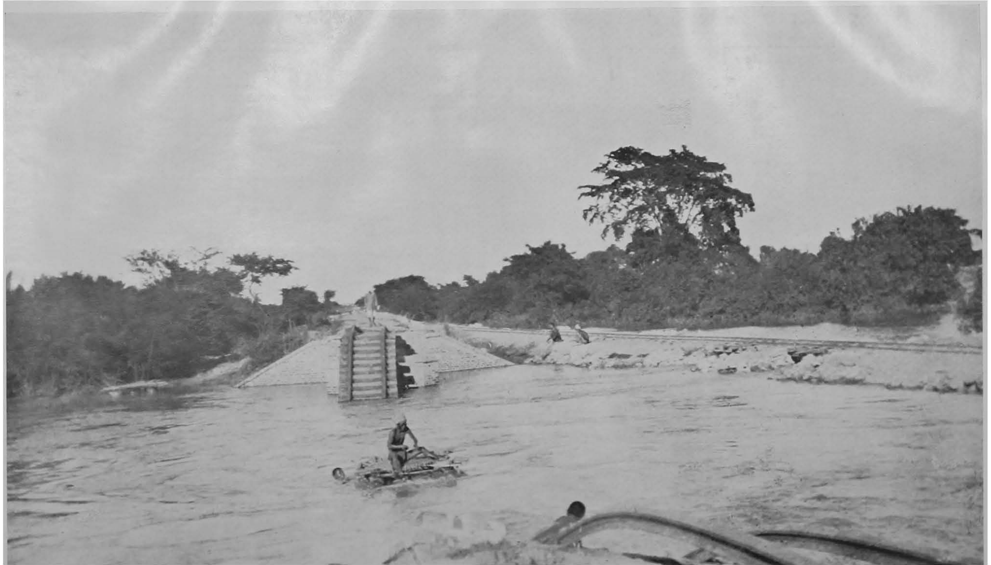
BREACH AT BRIDGE 192, MILE 335-1.
