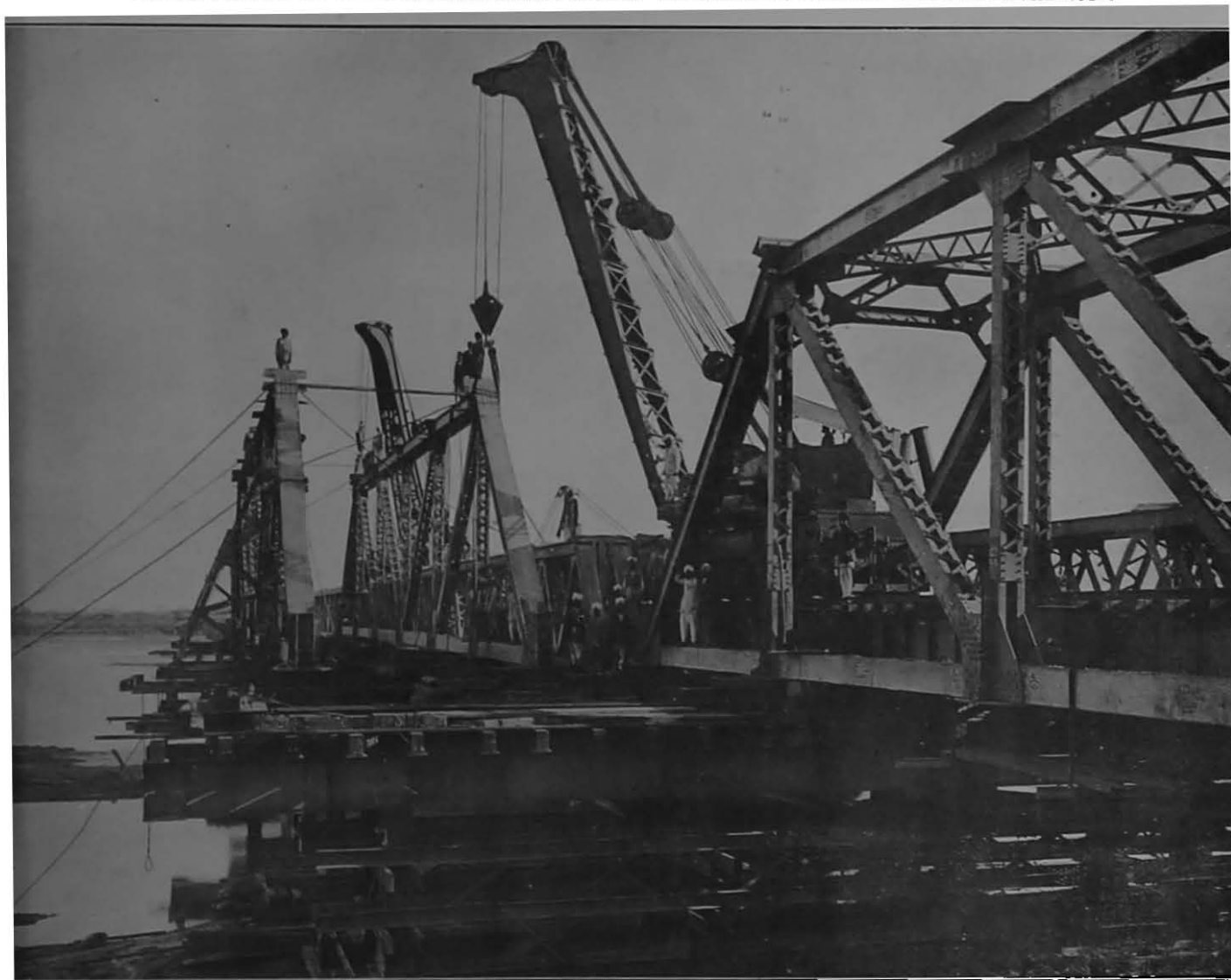
Girder of second span lowered into position on staging.
