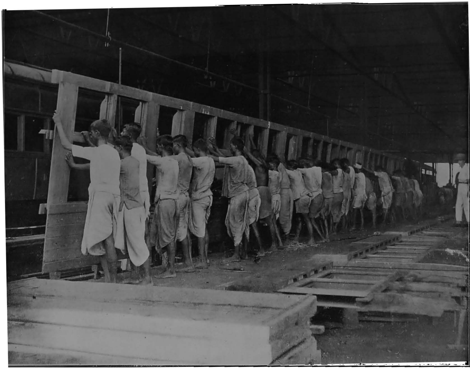
Progressive Carriage Building at Lilloah, East Indian Railway, showing a complete side of a carriage being lifted into position.
