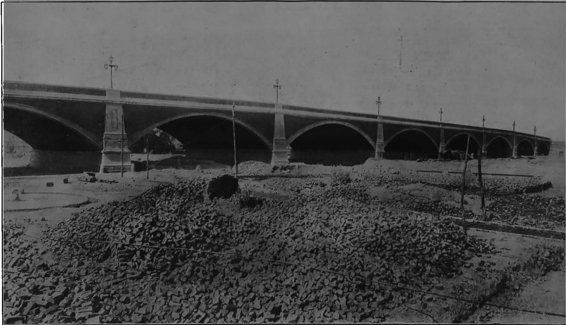
A view of the completed bridge.
