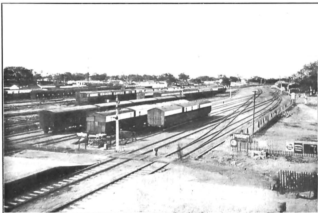
Secunderabad Station Yard.
