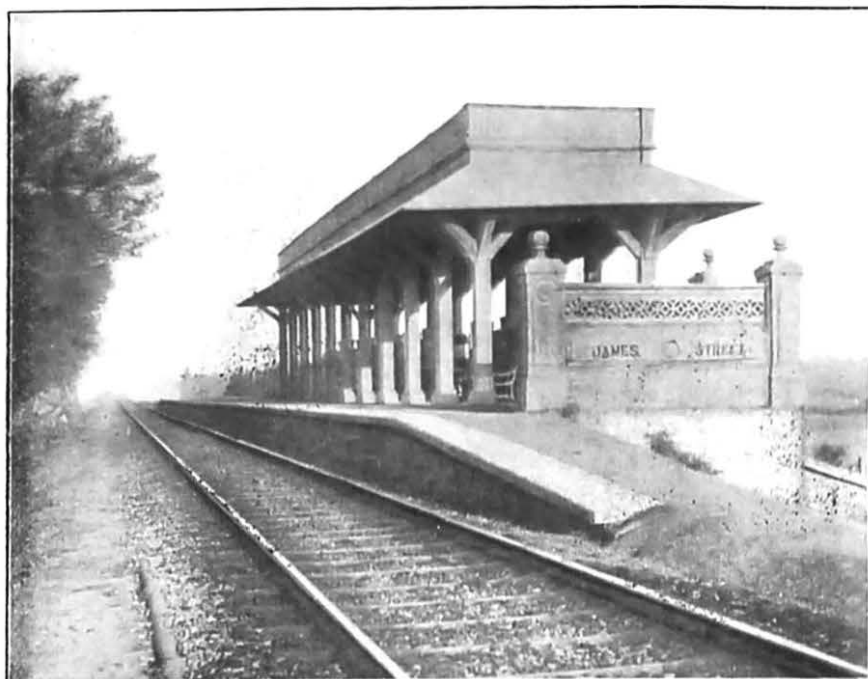
James Street Station, a suburban station recently rebuilt in reinforced concrete.
