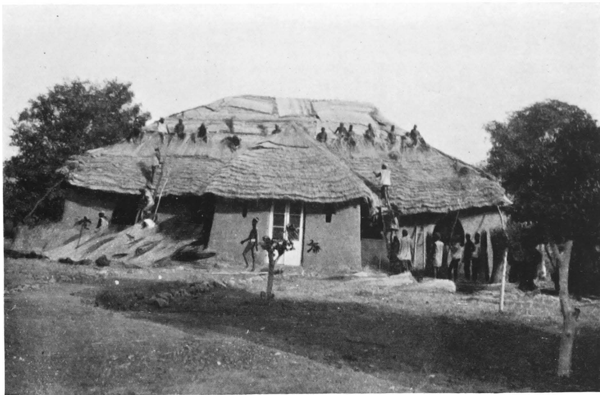
RE-ROOFING THE HOUSE
