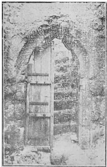
Fort Tunga : The Doorway, showing the precipitous flight of stonesteps.
