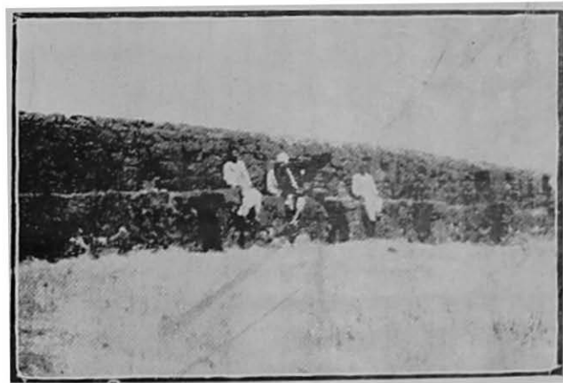
Prachandgad. A peculiar provision in one part of the parapet wall - supporting stone slabs jutting out of the rampart as rests for the archers or gunners.
