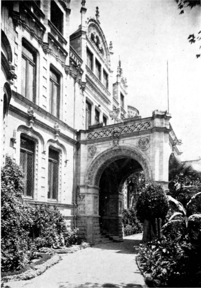
Some of the Private Residences in the Cities Are Very Large and Resemble Spacious Office Buildings. They Have a Large Patio in the Center of the Dwelling.
