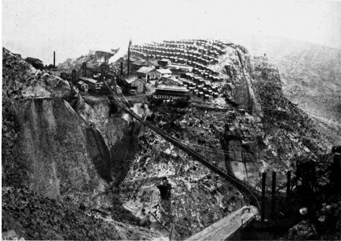
A Mine Near Durango. Notice the Small Huts on the Hillside for the Miners' Homes,
