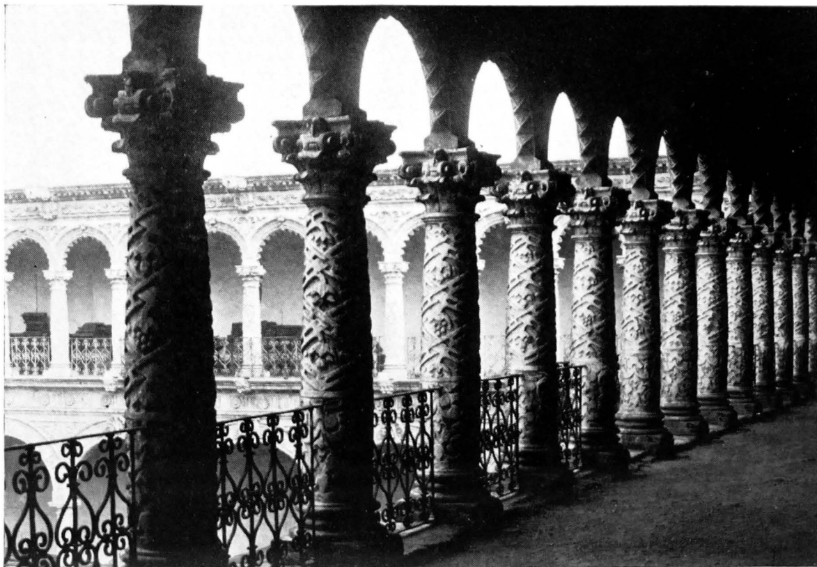
Within the Patio Balcony of the La Merced Convent, Mexico City.
