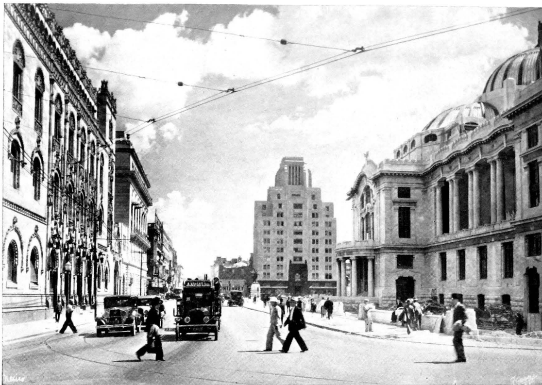
Teatro Nacional Street in Mexico City. Post Office and Bank of Mexico (on left) The National Theatre of Fine Arts (on right). In the Background One Can View Mexico's Only Skyscraper, Erected Upon Countless Pillings to Offset Sinking Such as Most All Other Large Buildings Have Experienced in the Capital City.
