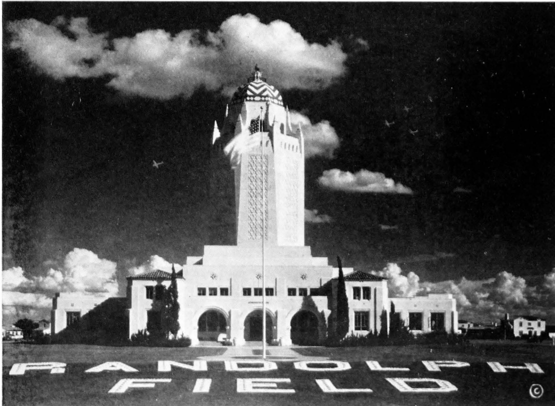
Administration Building, Randolph Field, San Antonio, Texas. San Antonio is Often Referred to as the "West Point" of the Air.
