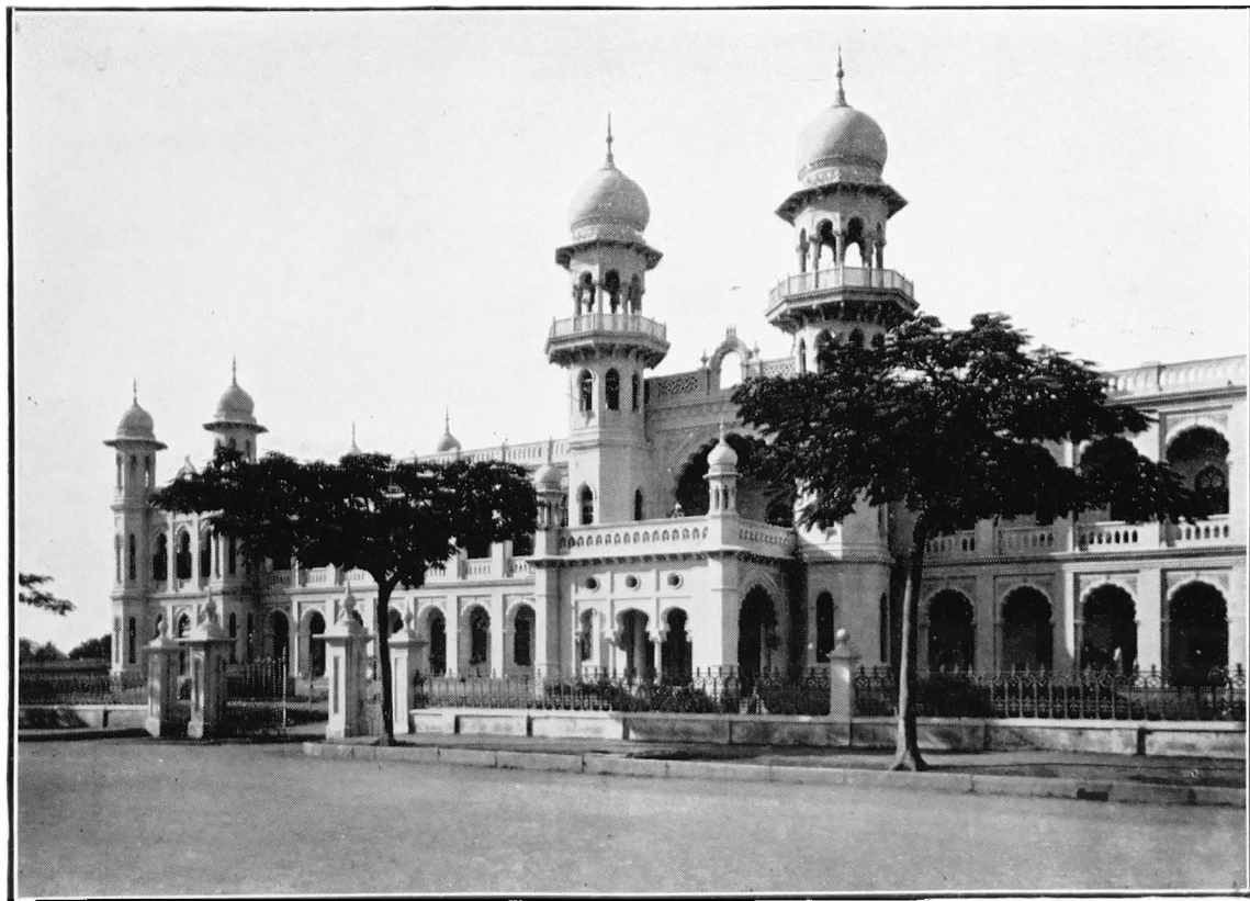
THE MUNICIPAL OFFICES, MYSORE
